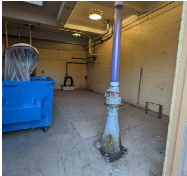
Figure 4: Bar Screen Sluice Gate
