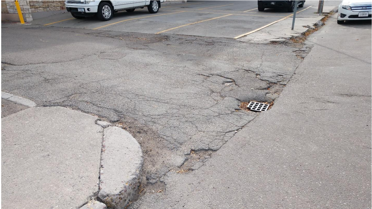
3 1 st Alley S, East Side. Location of inlet to be replaced
