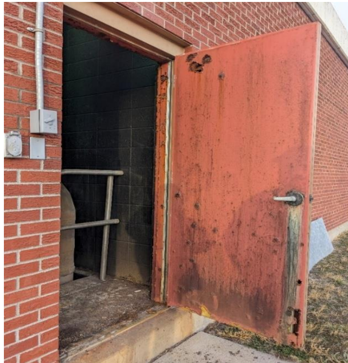
Figure 1: Corroded Door to Wet Well
