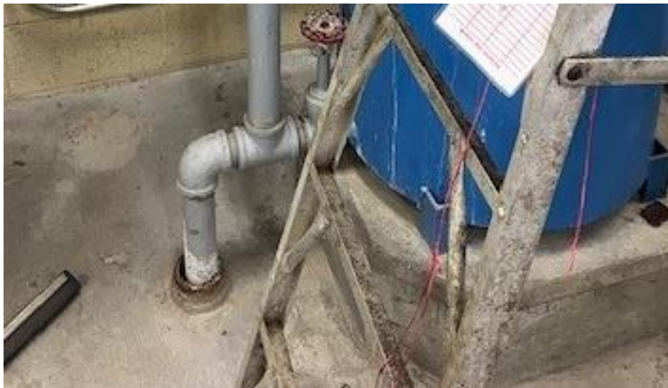
Figure 3: Corroded Drainpipe to Wet Well
