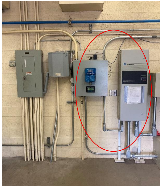
Figure 2: Single Non-operational VFD
