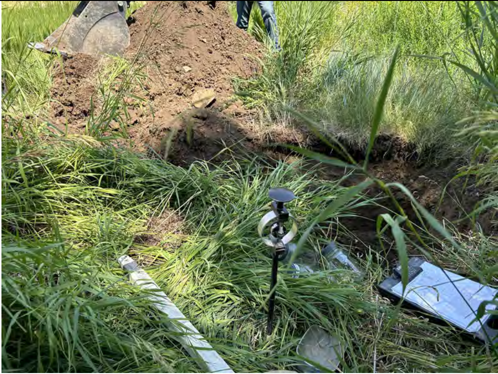
Description: TP-07 Cone penetrometer was pushed 4.25 inches under a 320 psi loading.
