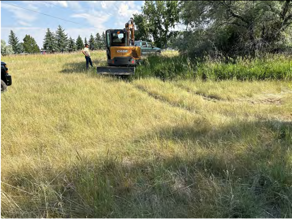
Description: TP-04 Location. View is to the south.
