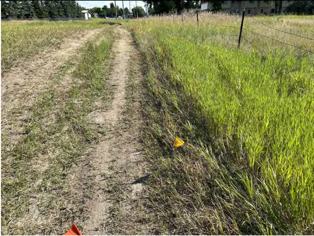
Description: Initial TP-04 area. Buried gas and communication utilities are indicated by pin flags.
