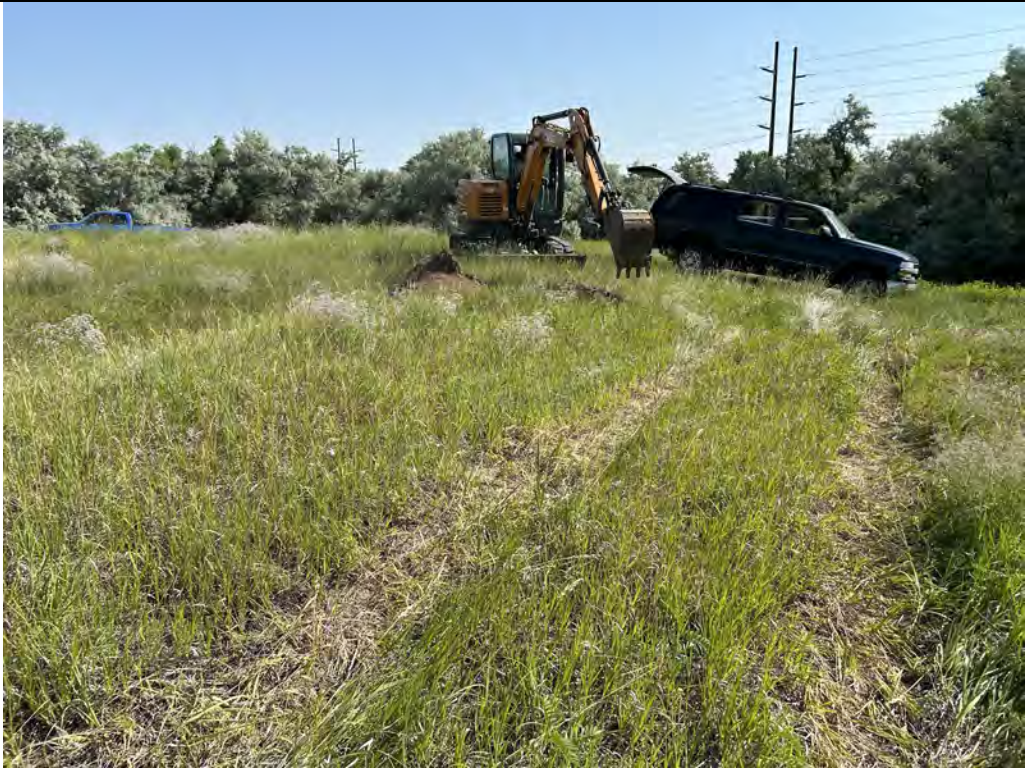
Description: TP-03 Location. View is to the north.
