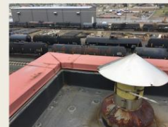
HVAC repairs on solids building ($1.1M)
