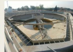
WWTP Final Clarifier Rehabilitation ($4.3M)
