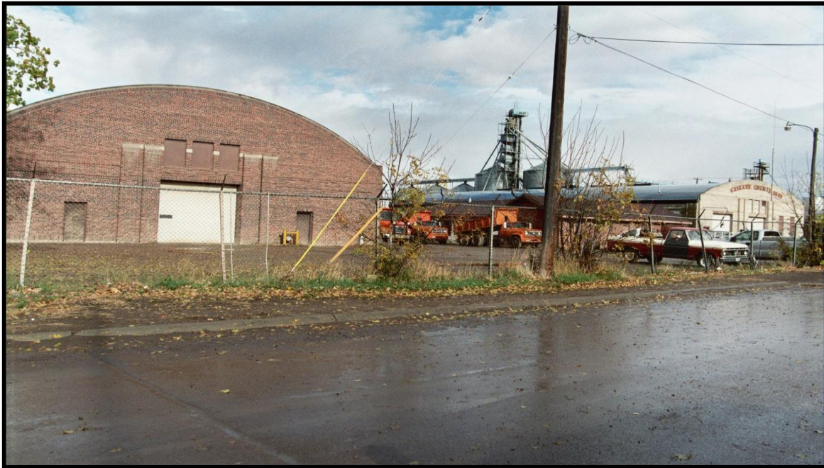
Figure 2 Cascade County Shops
