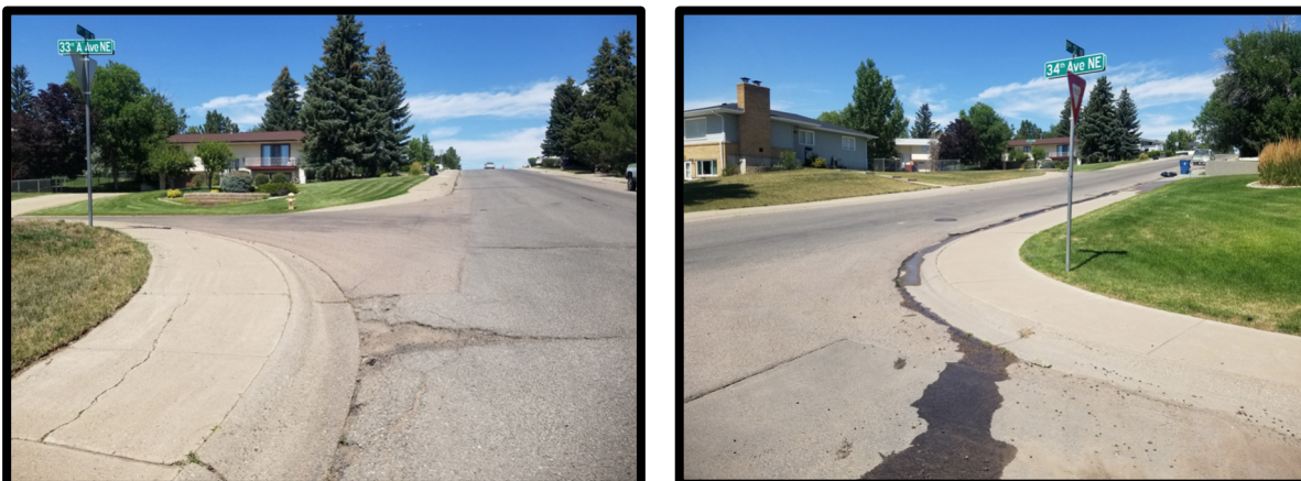
Lack of handicap ramps at intersection along project corridor. (Photos 07282025)
