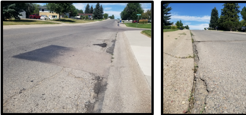
Existing damage to asphalt along 9 th St. NE from 32 Ave NE to 36 Ave NE. (Photos 07282025)
