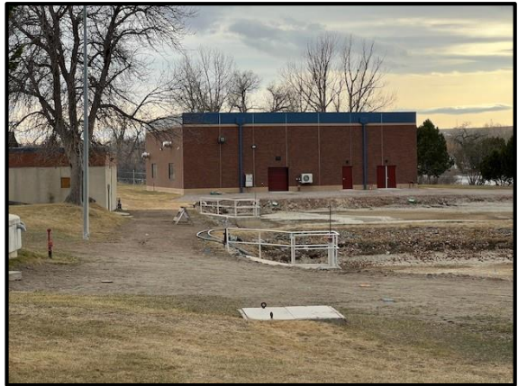
Solids Mitigation Building WTP
