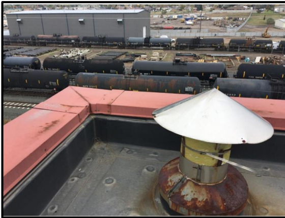
HVAC & Lighting Repairs on Solids Building
