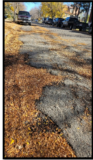
Existing damage to asphalt and curb along 4 th Ave North including non-standard storm inlet. (Photos 10222024)
