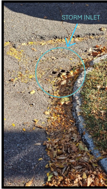
Existing damage to asphalt and curb along 4 th Ave North including non-standard storm inlet. (Photos 10222024)
