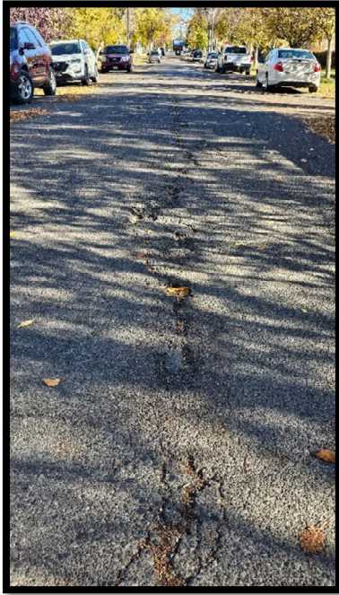
Existing damage to asphalt and curb along 4 th Ave North including non-standard storm inlet. (Photos 10222024)
