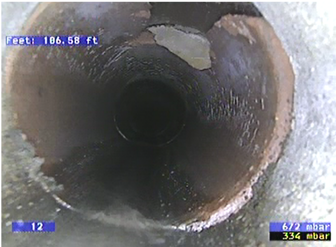
Figure 2 Existing 8" Clay pipe, Sanitary Sewer Main installed 1958
