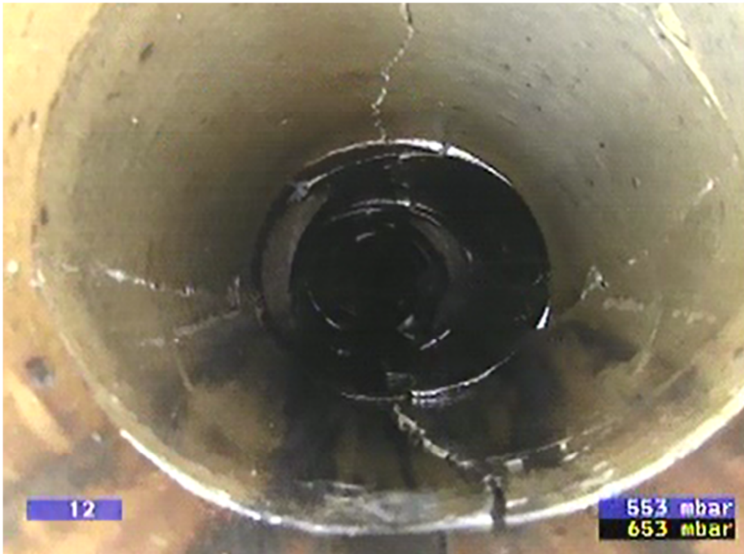
Figure 1 Existing 9" Clay pipe, Sanitary Sewer Main installed 1890
