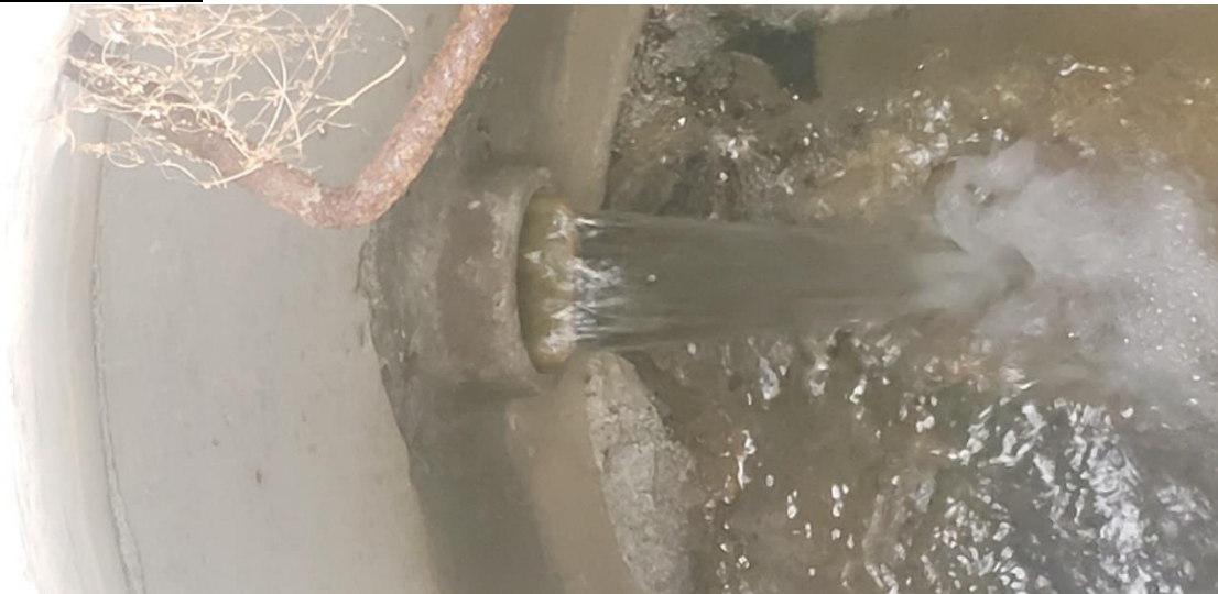
Figure 1 Foundation drain, approximately 50 gpm
