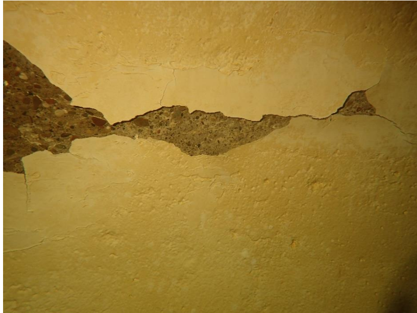
Figure 2 Cracks and flaking inside of tank
