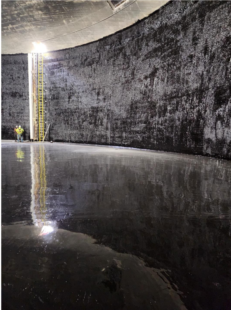
Figure 5 Inside of tank with the liner installed
