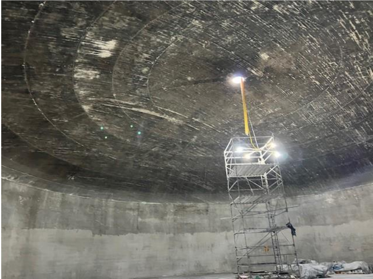
Figure 4 Inside of tank during cleaning
