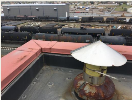
HVAC repairs on solids building ($1.1M)
