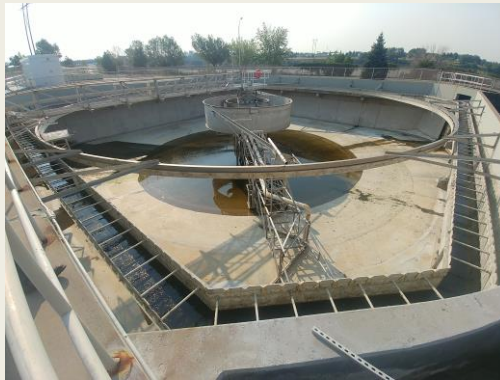
WWTP Final Clarifier Rehabilitation($4.3M)
