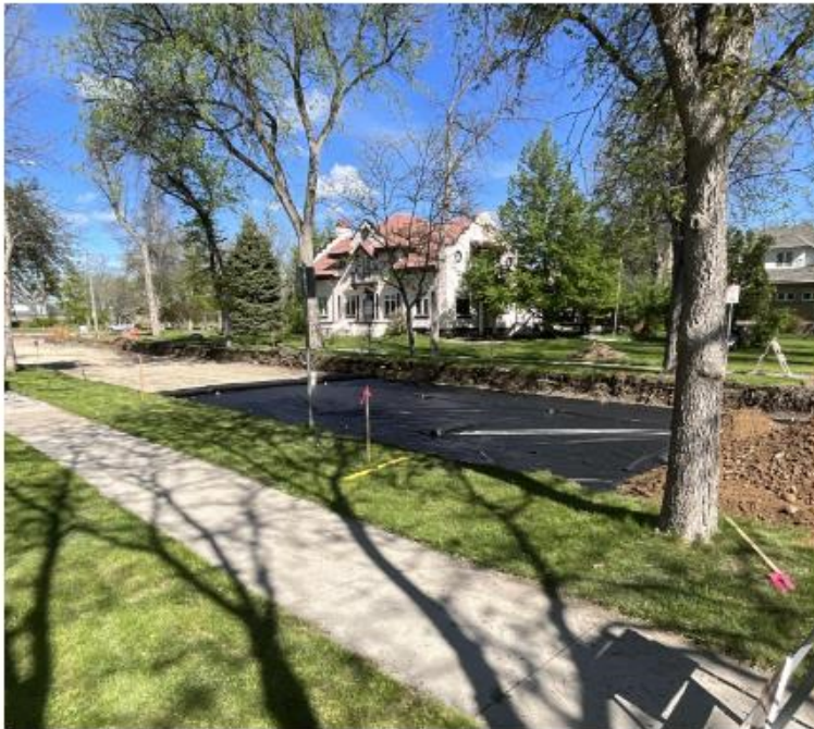
Fabric being placed over excavated subgrade
