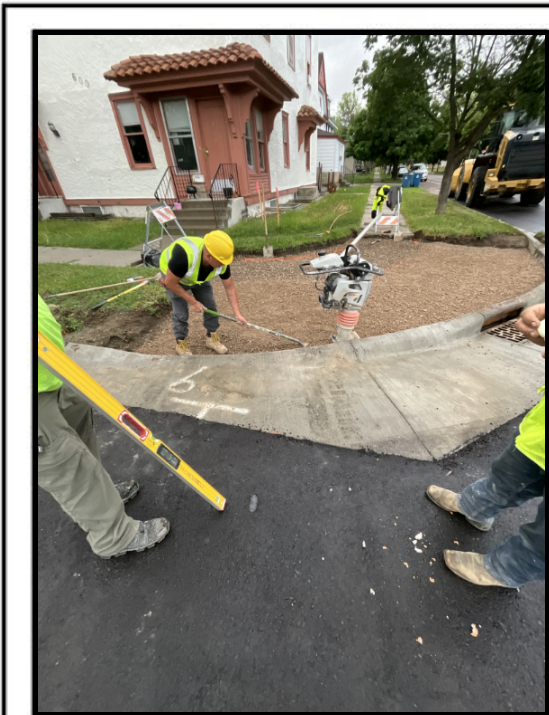
7th Ave N. & 6th St. N - Handicap Ramp Prep
