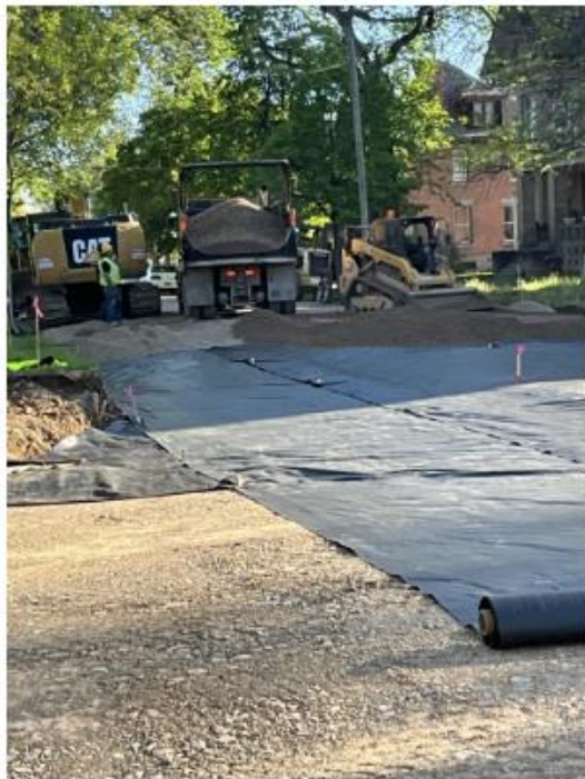
Fabric being placed over 8-inch sub-base
