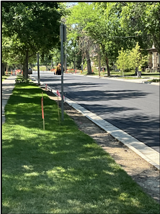
3rd Ave N. & 3rd St. N. (looking west) - Paving
