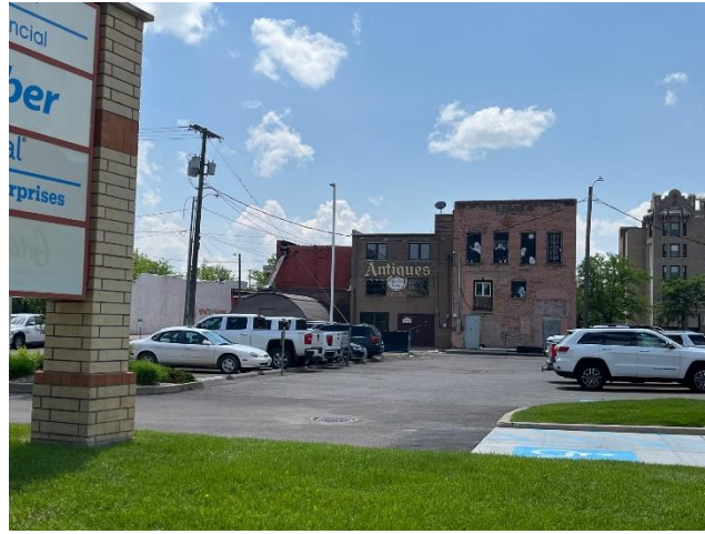
Image 03: Rear Façade view from 2 nd Ave N
