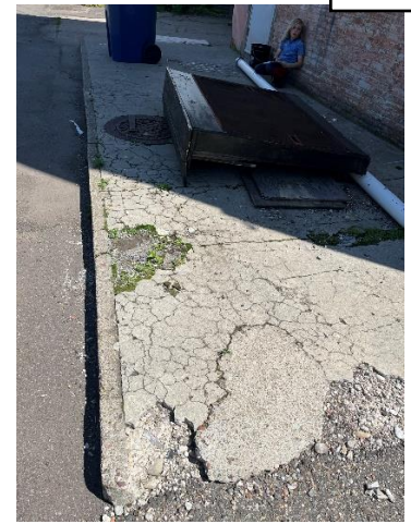
Image 04: Rear concrete slab
