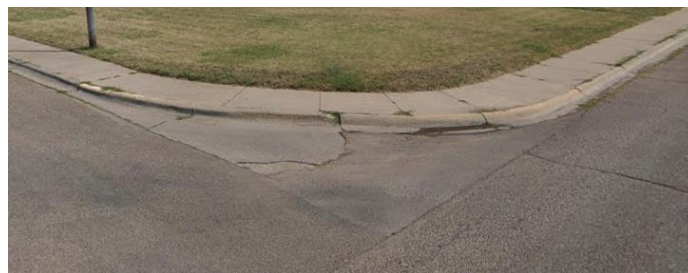
SE Corner of 32 nd St S and 5 th Ave S
