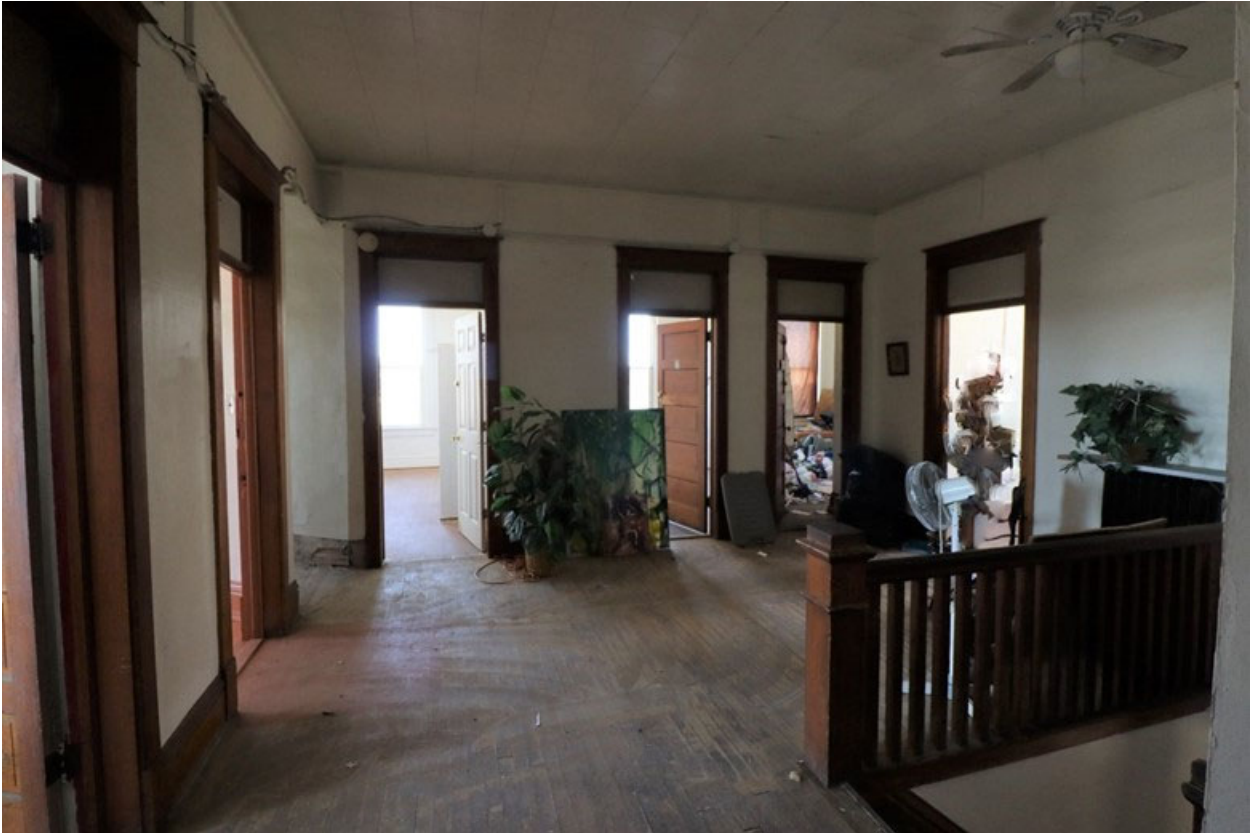
MT_CascadeCounty_BaatzBlock_0027: 3 rd floor lobby with top of original open stair in foreground showing original door locations and stained wood trim and base, original wood floors, July 1, 2021, looking north, photographer: Katie Batterbee.
