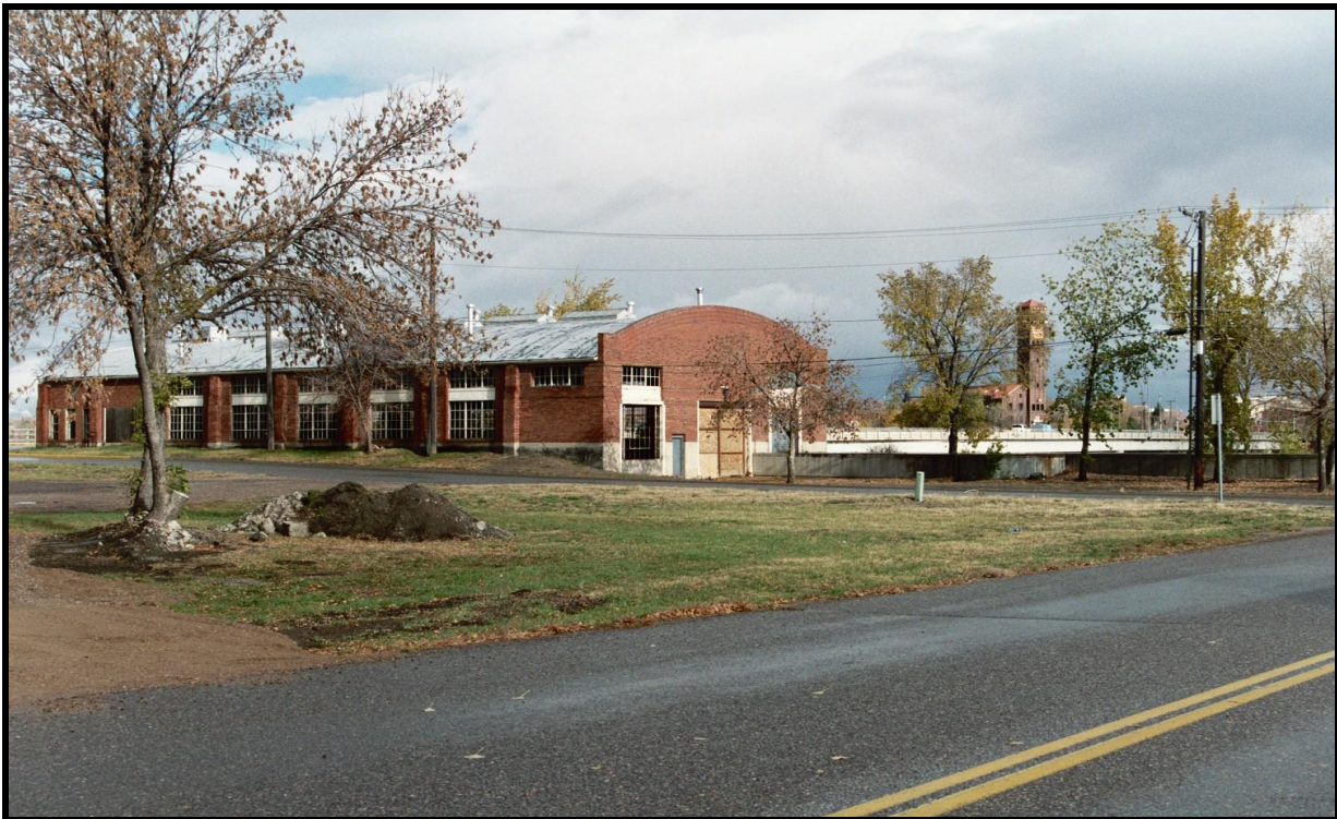
Figure 4. Former Highway Department Building
