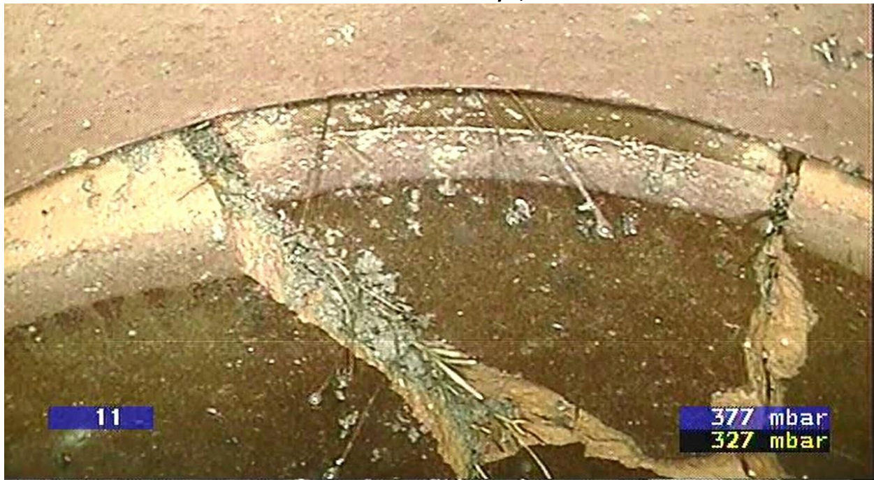
9" clay tile sewer main with a fracture.
