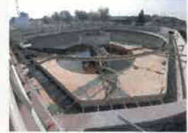
WWTP Final Clarifier Rehabilitation($4.3M)
