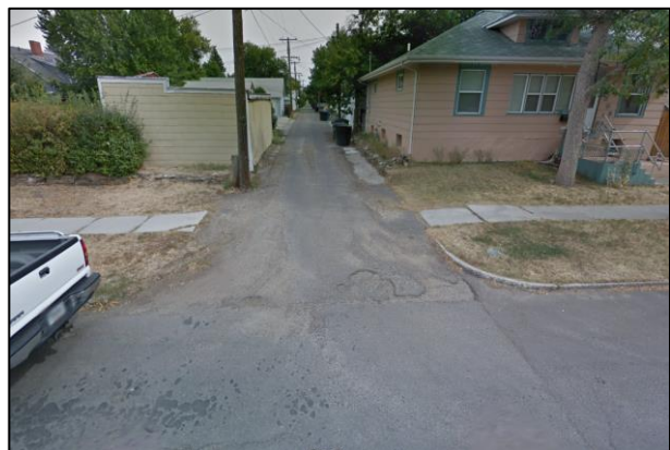
Ramps located at Alley Aprons
