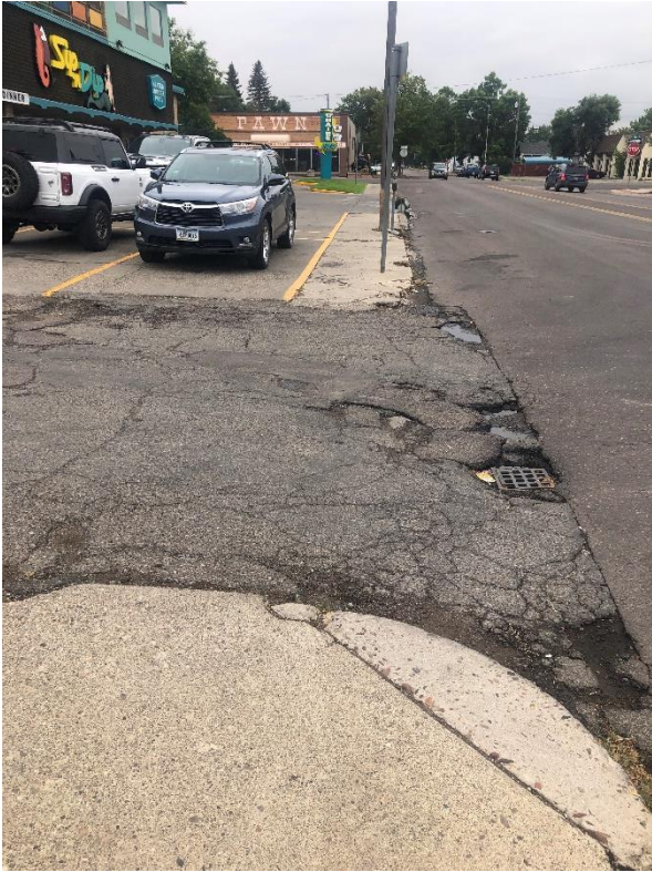
Alley, looking South
