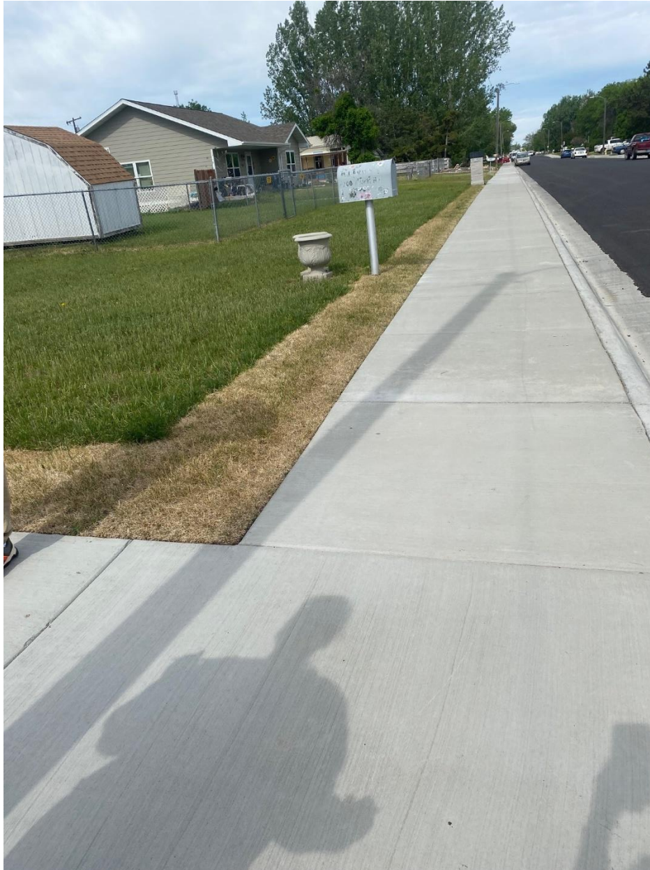
New sidewalk and road surface from Phase 1, 7th Ave NW at 12th St NW
