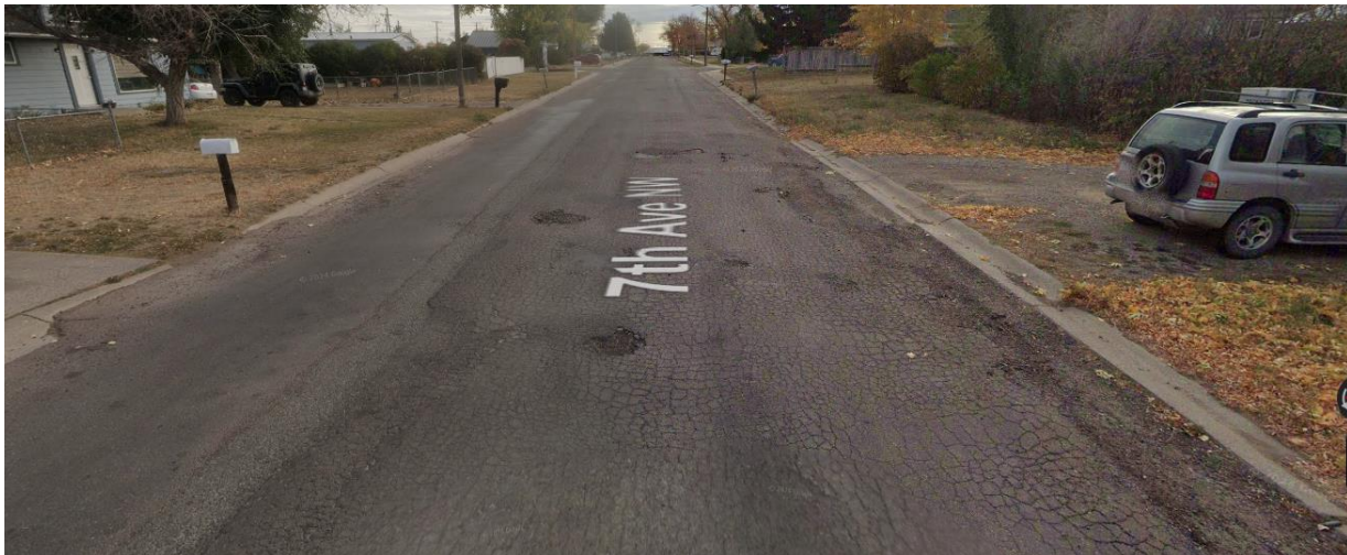
Mid block 7th Ave NW facing towards 11th St NW
