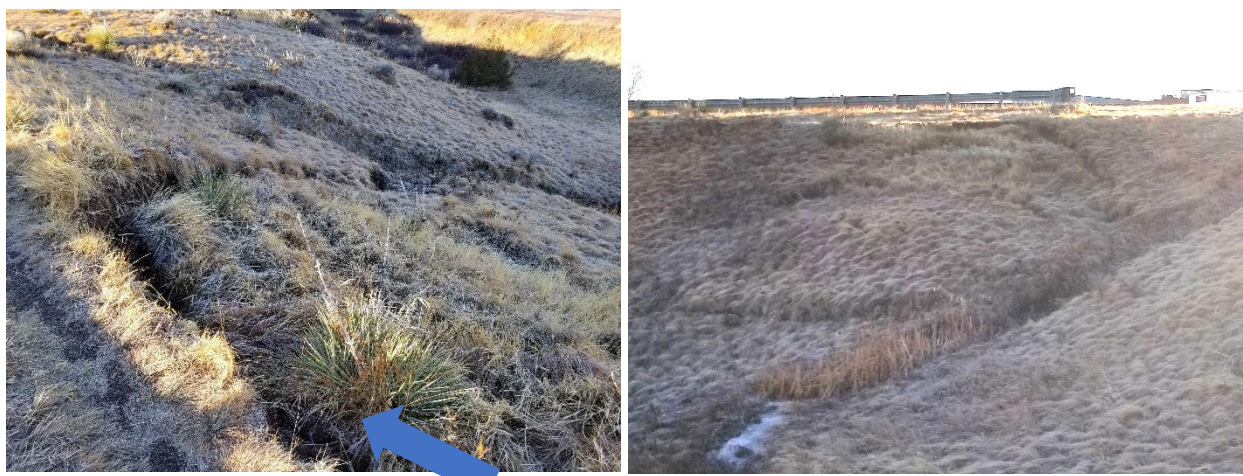
Fault/Separation Line in Soil
