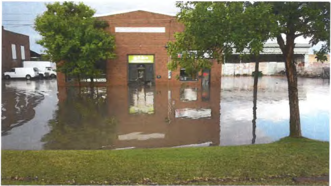
Builders Exchange Flooding (8-9-16)
