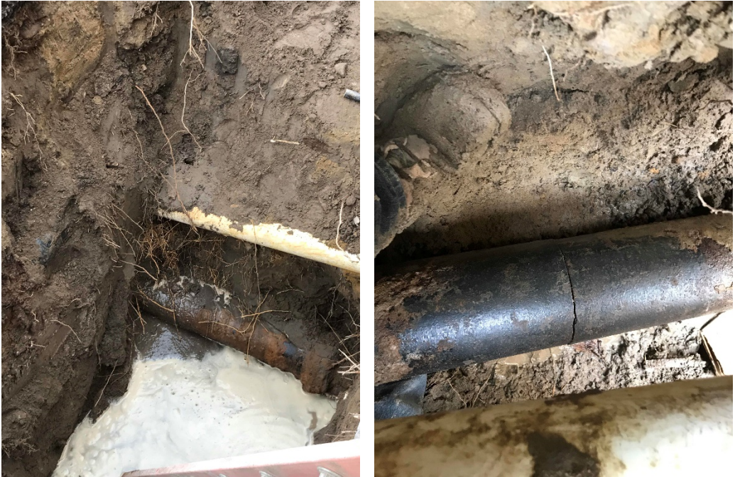
Station 3+35 (3 rd St S) Repair ruptured fire line
