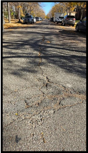
Existing damage to asphalt, curb, and handicap ramps along 4 th Ave North. (Photos 10222024)
