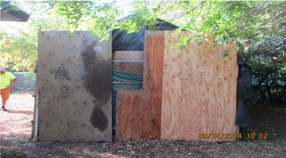
Secured temporary shelter
