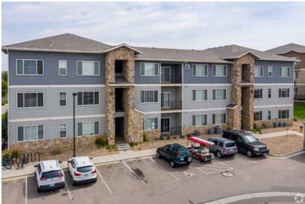
Creek View Apartments, Greeley, CO
