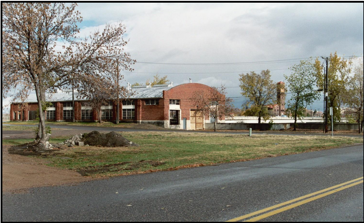
Figure 4. Former Highway Department Building
