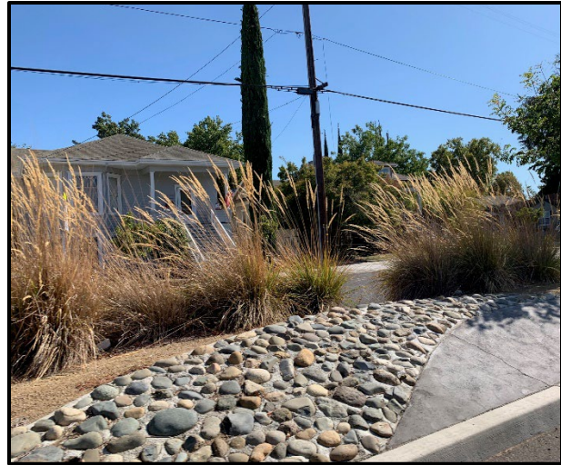
Installed median landscape with concrete, cobble, planting
