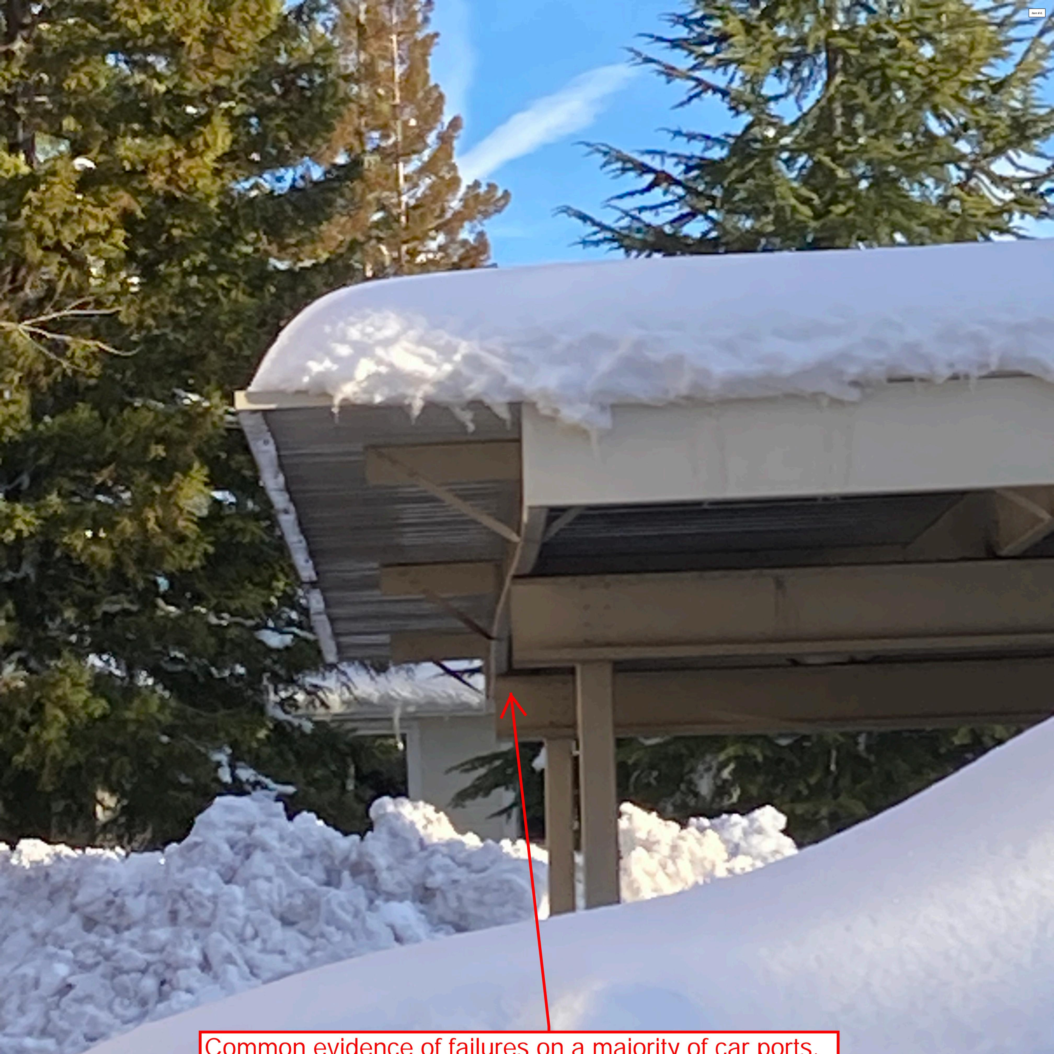
Common evidence of failures on a majority of car ports. Structural steel twisting due to snow load.
