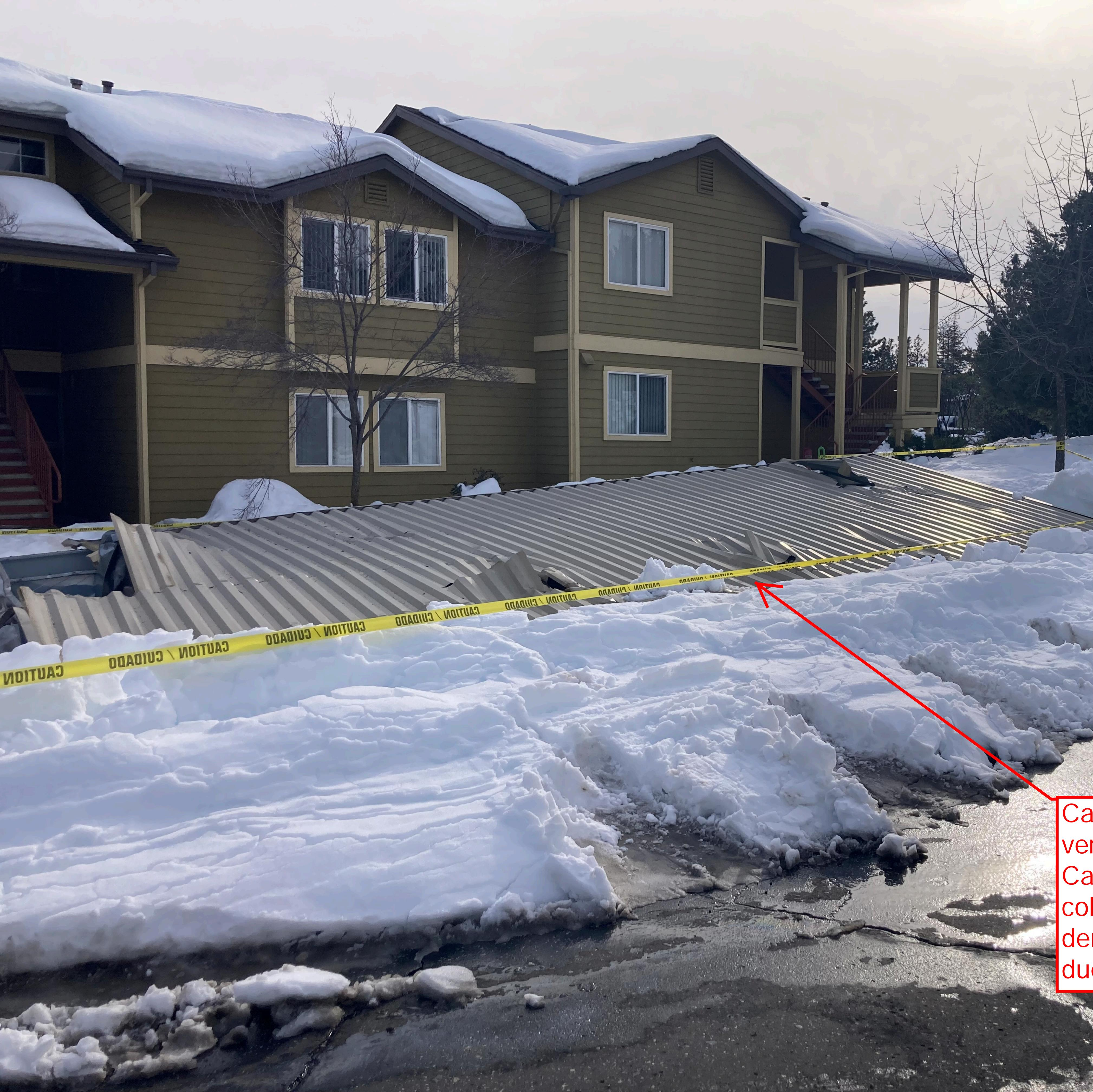
Catastrophic failure of vertical structural members. Carport was partially collapsed and was demolished immediately due to tenant safety. ltem # 6.
