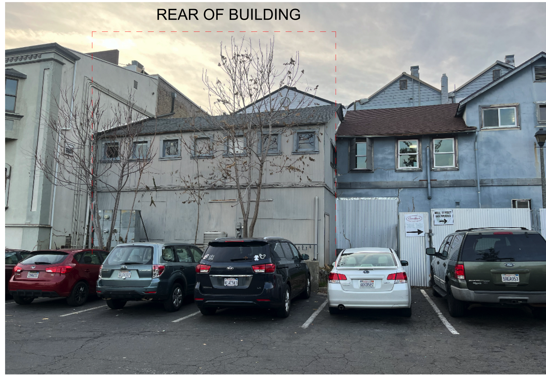
145 MILL STREET VIEW - REAR OF BUILDING
