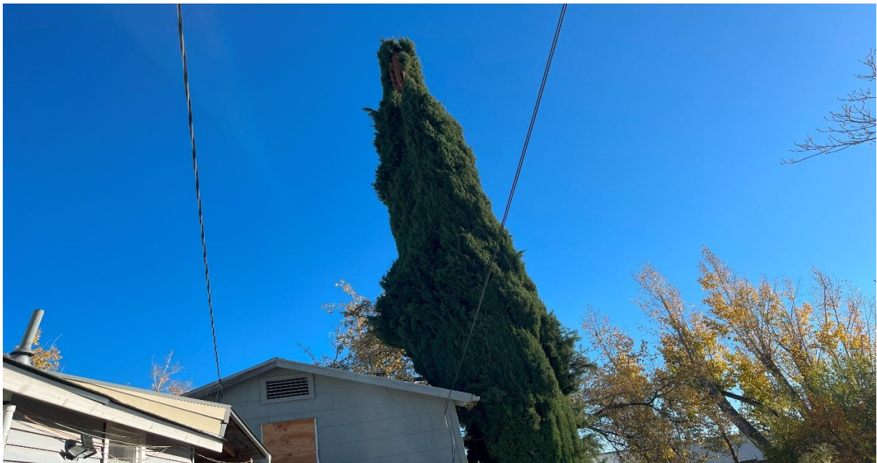
Photo 2: The existing large non-native tree along the parcel border is a hazard tree given it is a fire danger and a danger to infrastructure within the subject parcel.
