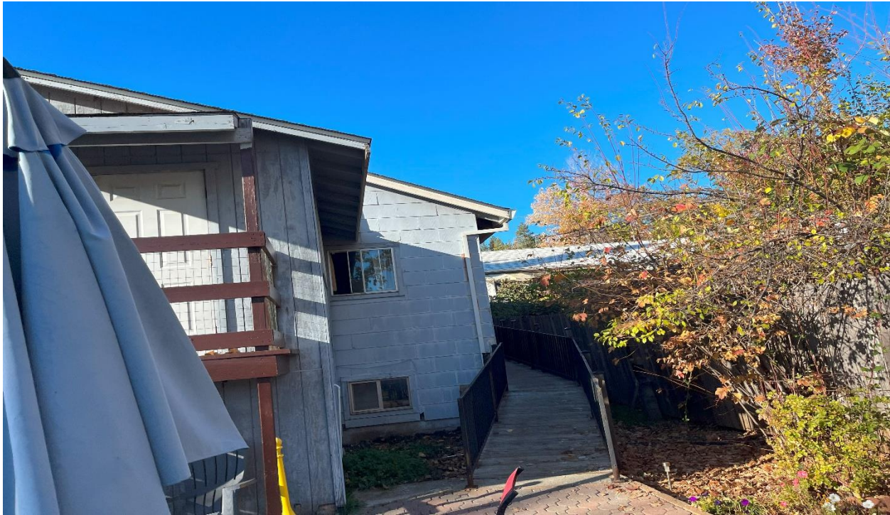
Photo 10: Far side of the subject parcel with no native trees or encroachment of trees within the parcel.
