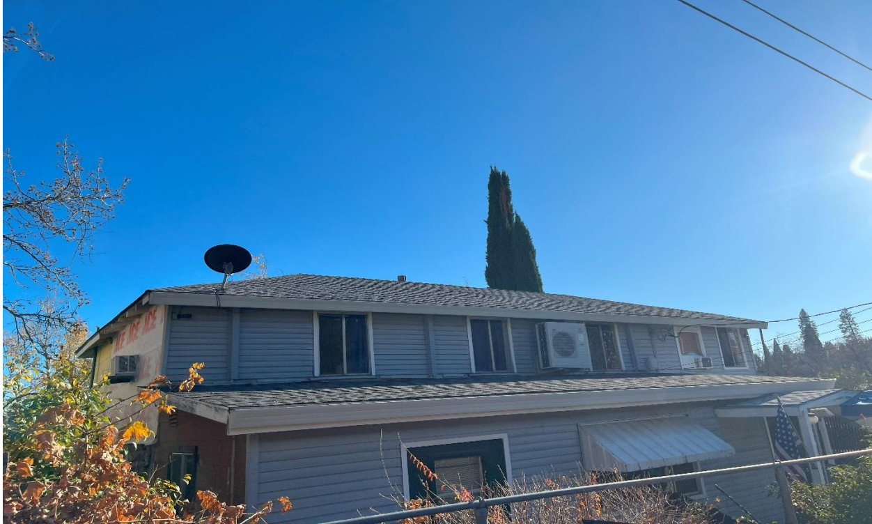
Photo 9: Existing structure within the subject parcel from along Glenwood Avenue. Only the tall non-native tree in photo and the blue oak tree encroach within the parcel.
