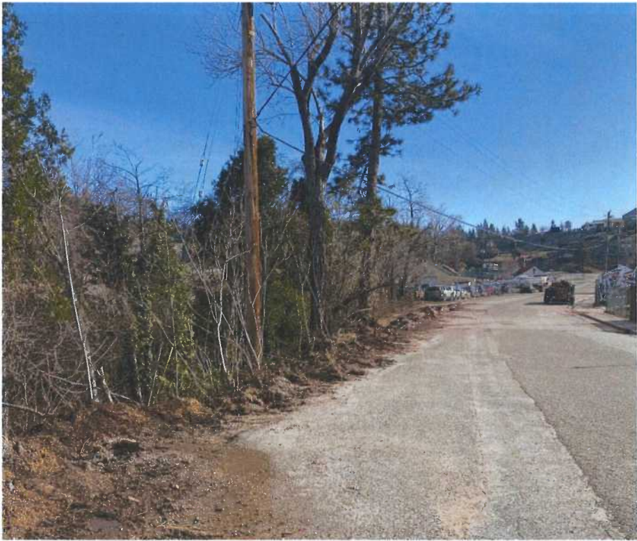
Photo 6: Representative Photo of Segment 4 along Railroad Ave. facing northeast. The proposed trail runs down the center of the image along left side of the road, including road shoulder and graveled area. Wolf Creek in left of image.
