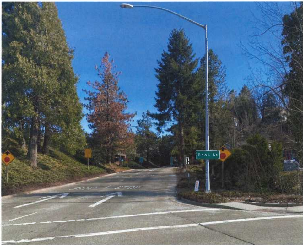
Photo 4: Representative Photo of Segment 3 facing northeast. The proposed trail location is down the center of the image including portion of the right side of the existing road, right shoulder, and some of landscaped area.
