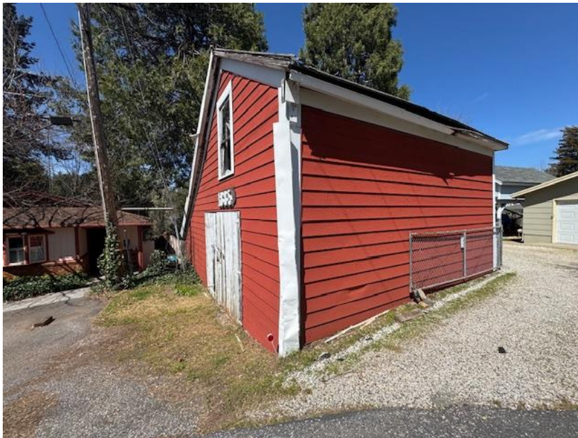
Photograph 2: View looking northwest at the southeast elevation of the barn. Note that the siding on these two elevations is aluminum clapboards.
