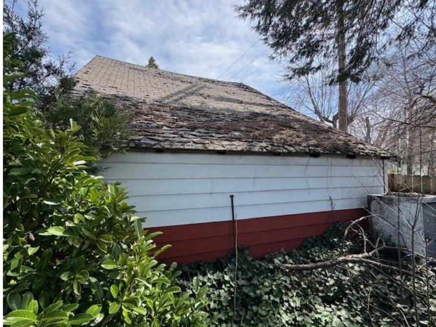
Photograph 5: View of the west elevation that has been reconstructed with plywood and aluminum clapboards.
