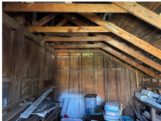
Photograph 12: View looking at the westernmost portion of the barn showing an original mortise and tenon wall on the left and a rebuilt wall on the south and the west.
