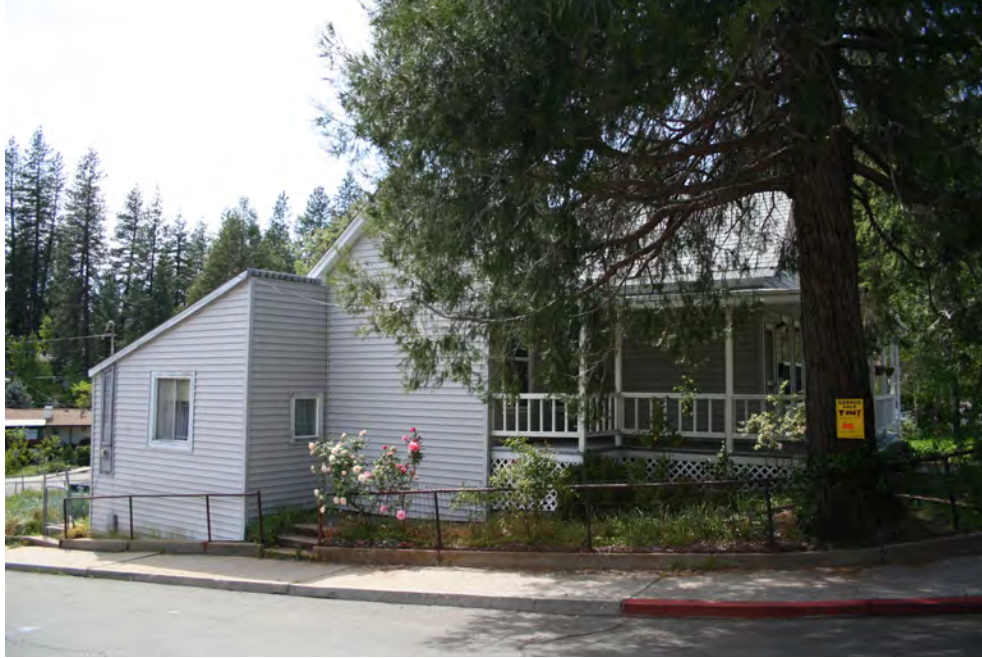
View looking southwest at the residence. Note the shed roof addition in the rear.
