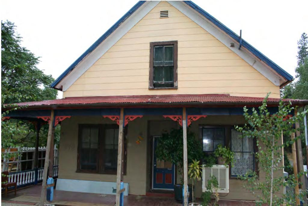
Close-up of the front facade of the residence. Note the bracing on the porch columns.
