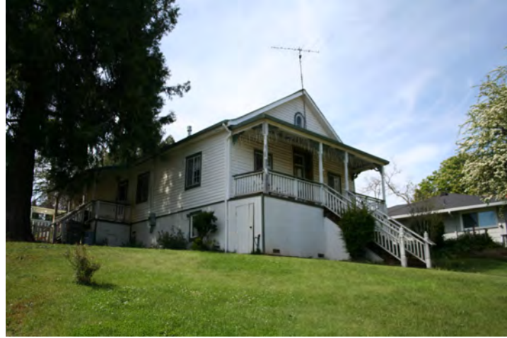
P5. Photograph or Drawing (Photograph required for buildings, structures, and objects.)
