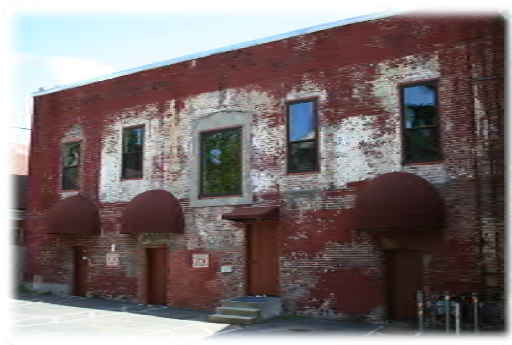
Replacement windows in a circa 1850s historic brick commercial building.
