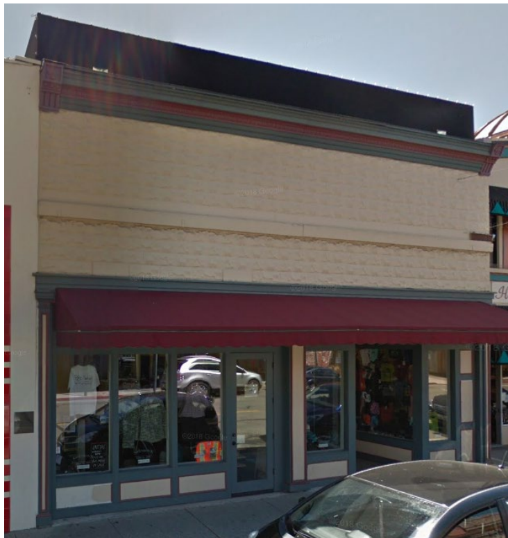
Existing storefront façade
