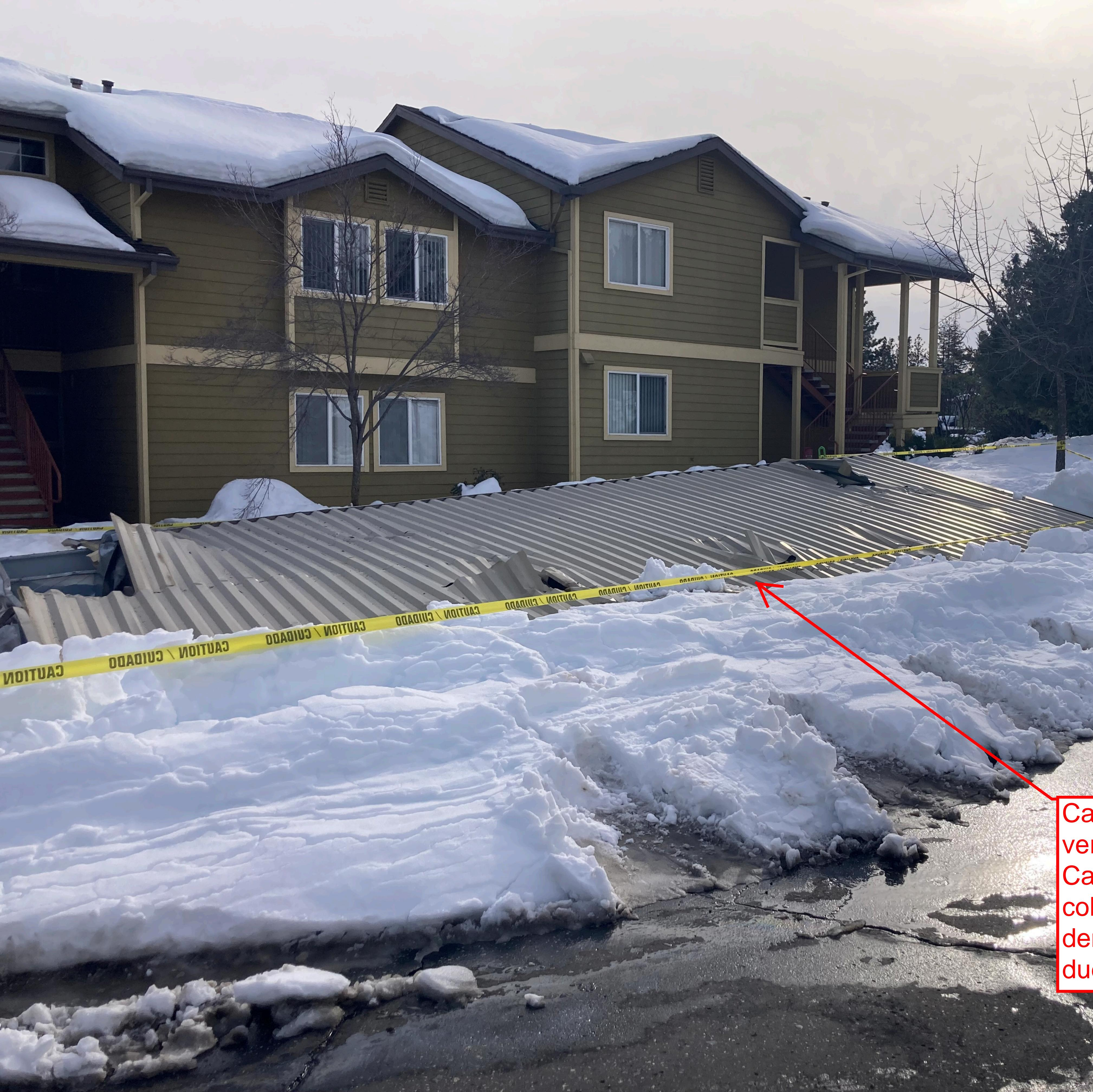
Catastrophic failure of vertical structural members. Carport was partially collapsed and was demolished immediately due to tenant safety. ltem # 2.
