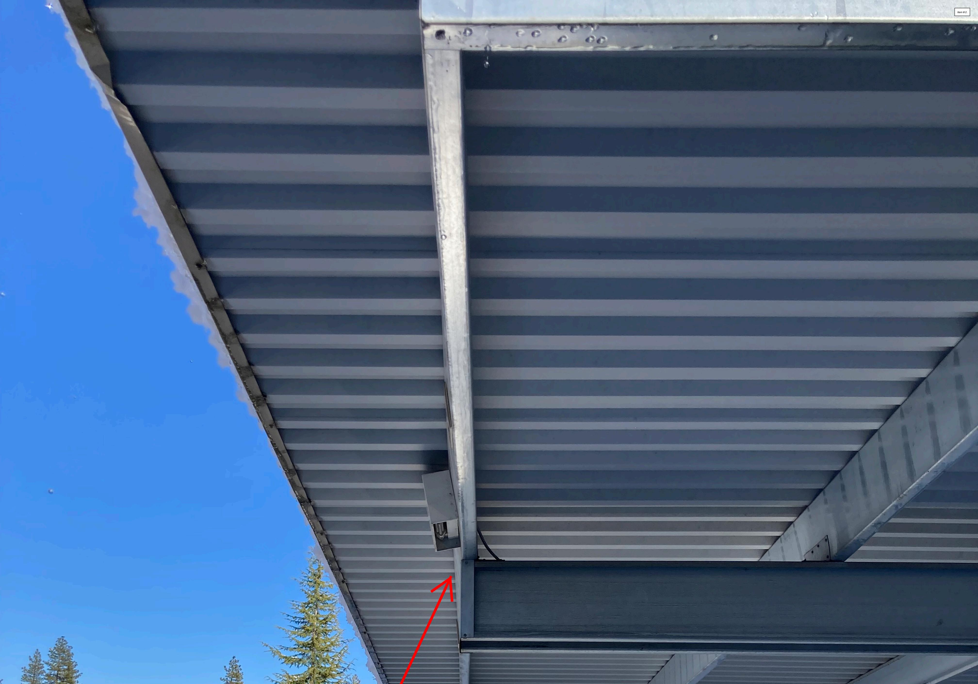
Structural members twisting due to snow load. This type of failure was typical throughout.
