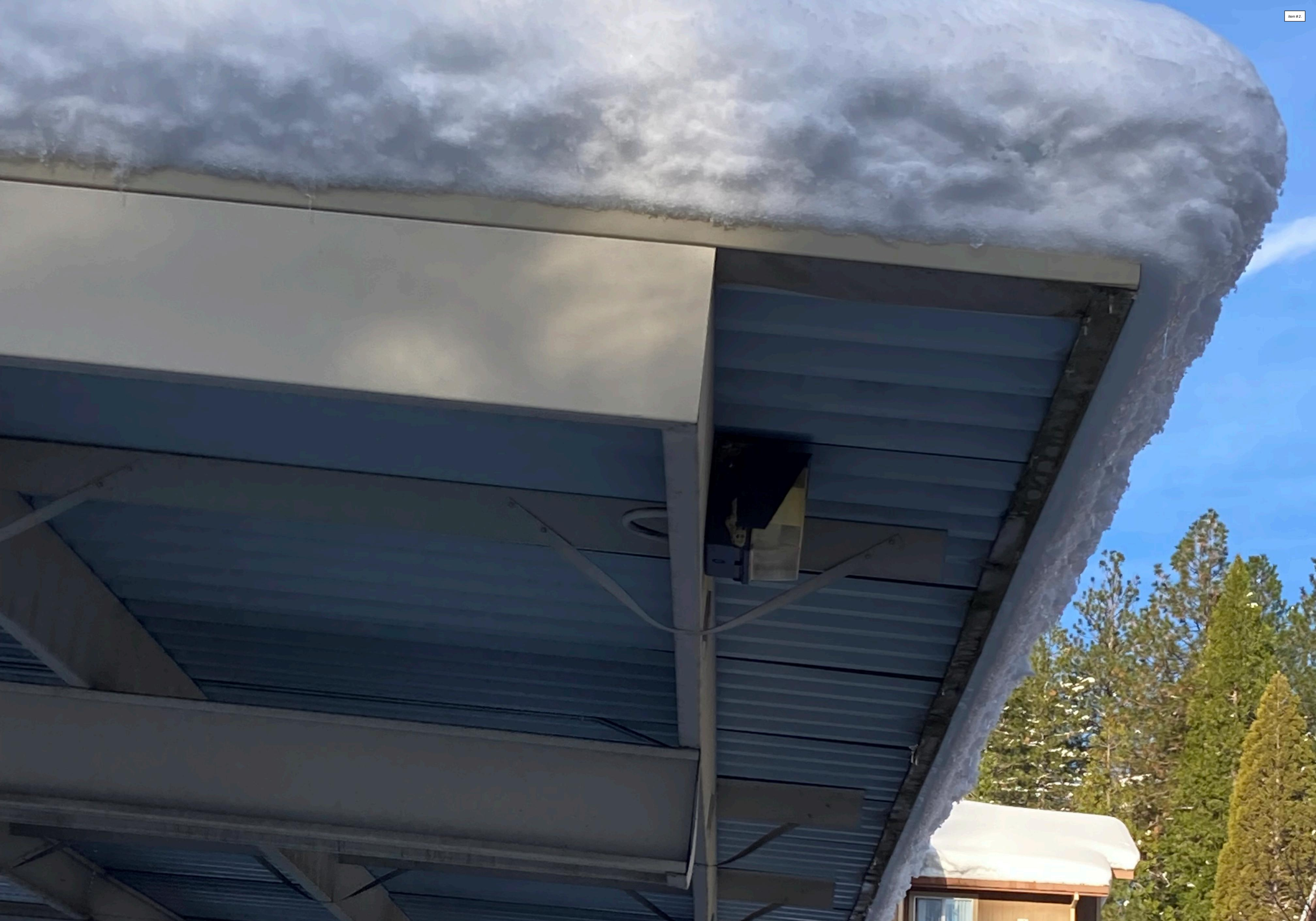
Twisting of structural member. Additionally, this carport is beginning to collapse from snow load. It is heavily tilted forward due to the weight of the snow and vertical columns weakening.
