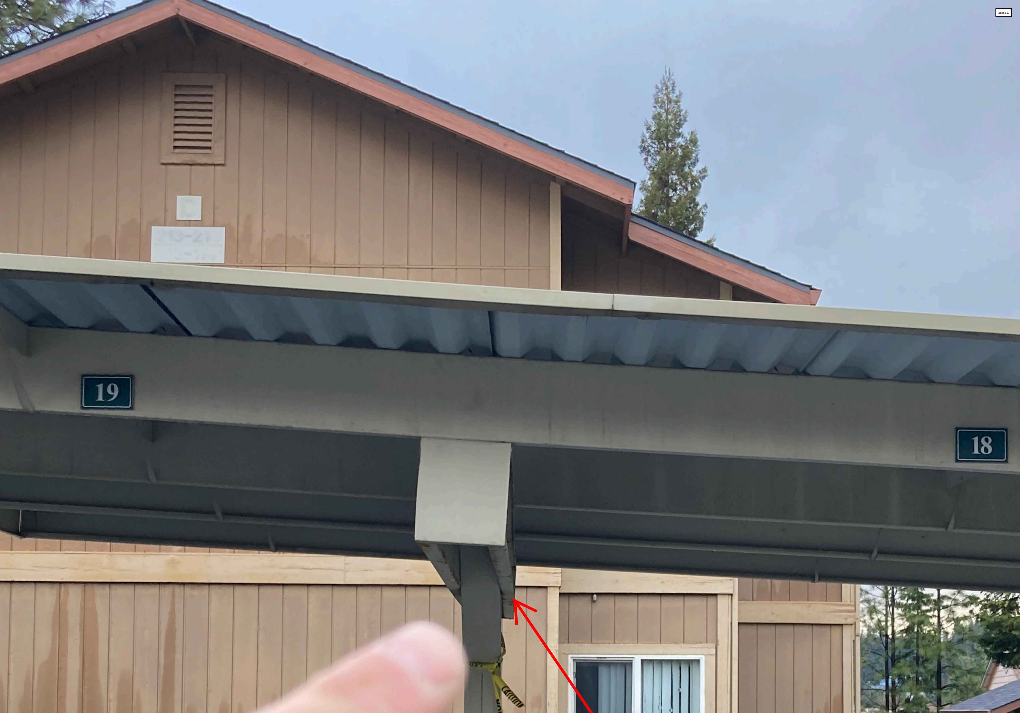
Beginning stage of failure at structural steel. This shows buckling at the mechanical connections of the cantilevered portion of the structural members.
