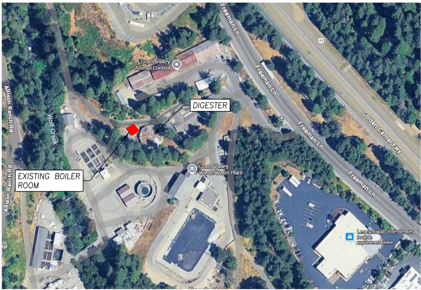
WASTEWATER TREATMENT PLANT 556 FREEMAN LANE
