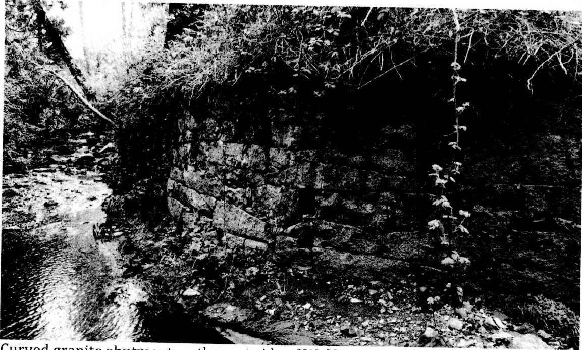
Curved granite abutment on the east side of Wolf creek viewed from the western bank. When the railroad grade constructed in 1875 followed the route of the creek with wooden approaches and dirt fill. Subsequent winter storm damage led the railroad to reinforce the trestle abutments with granite here.
