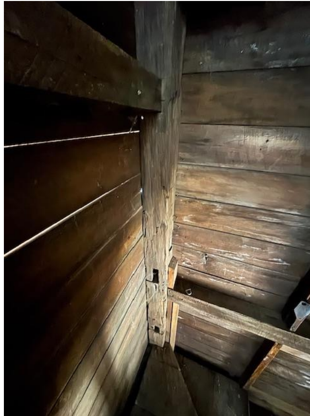
Photograph 11: View looking at the northeast corner of the lower floor wall showing a repurposed mortise and tenon beam.
