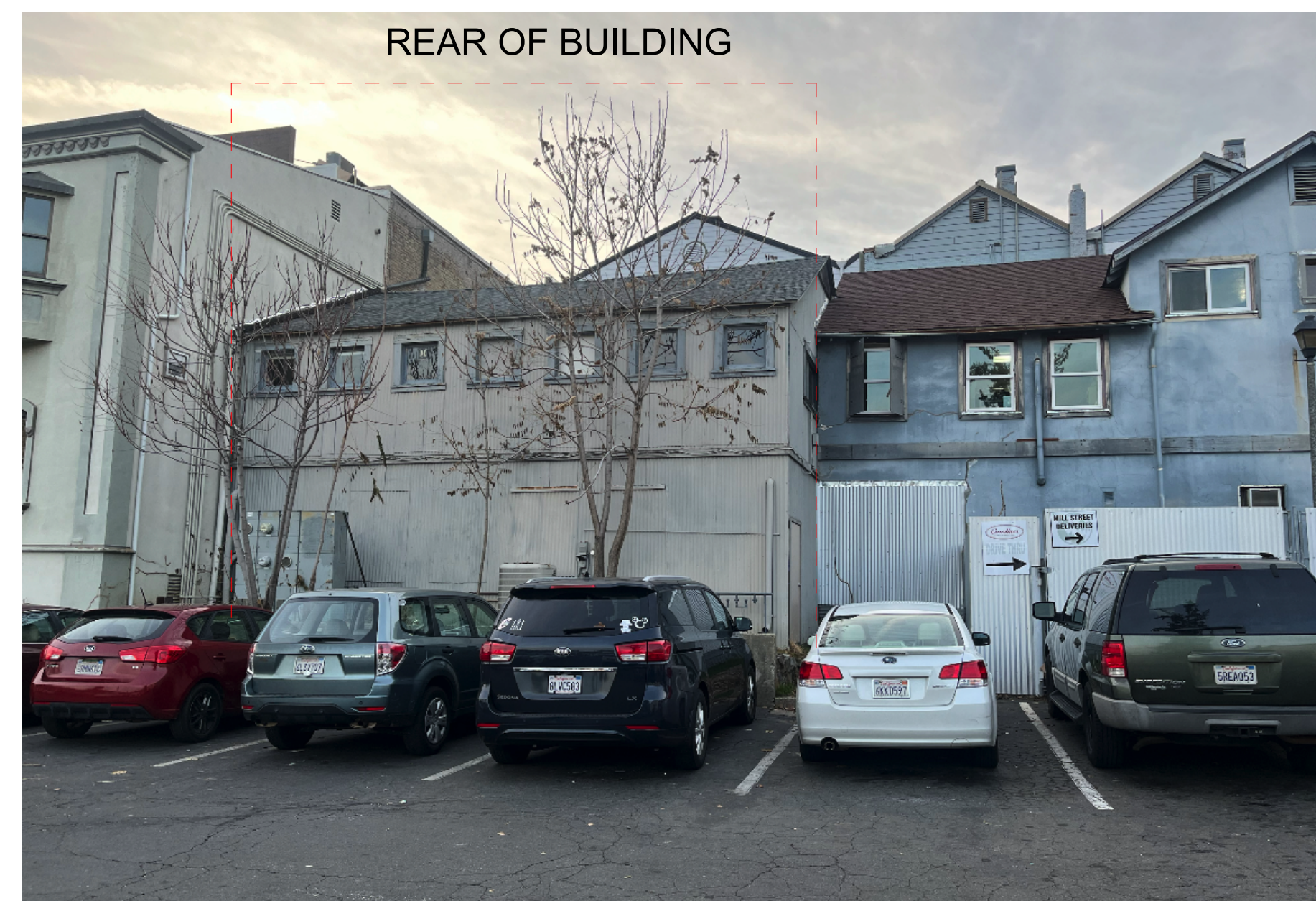
145 MILL STREET VIEW - REAR OF BUILDING
