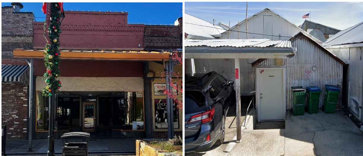
Existing Front and Rear Facades of 130 Mill Street
