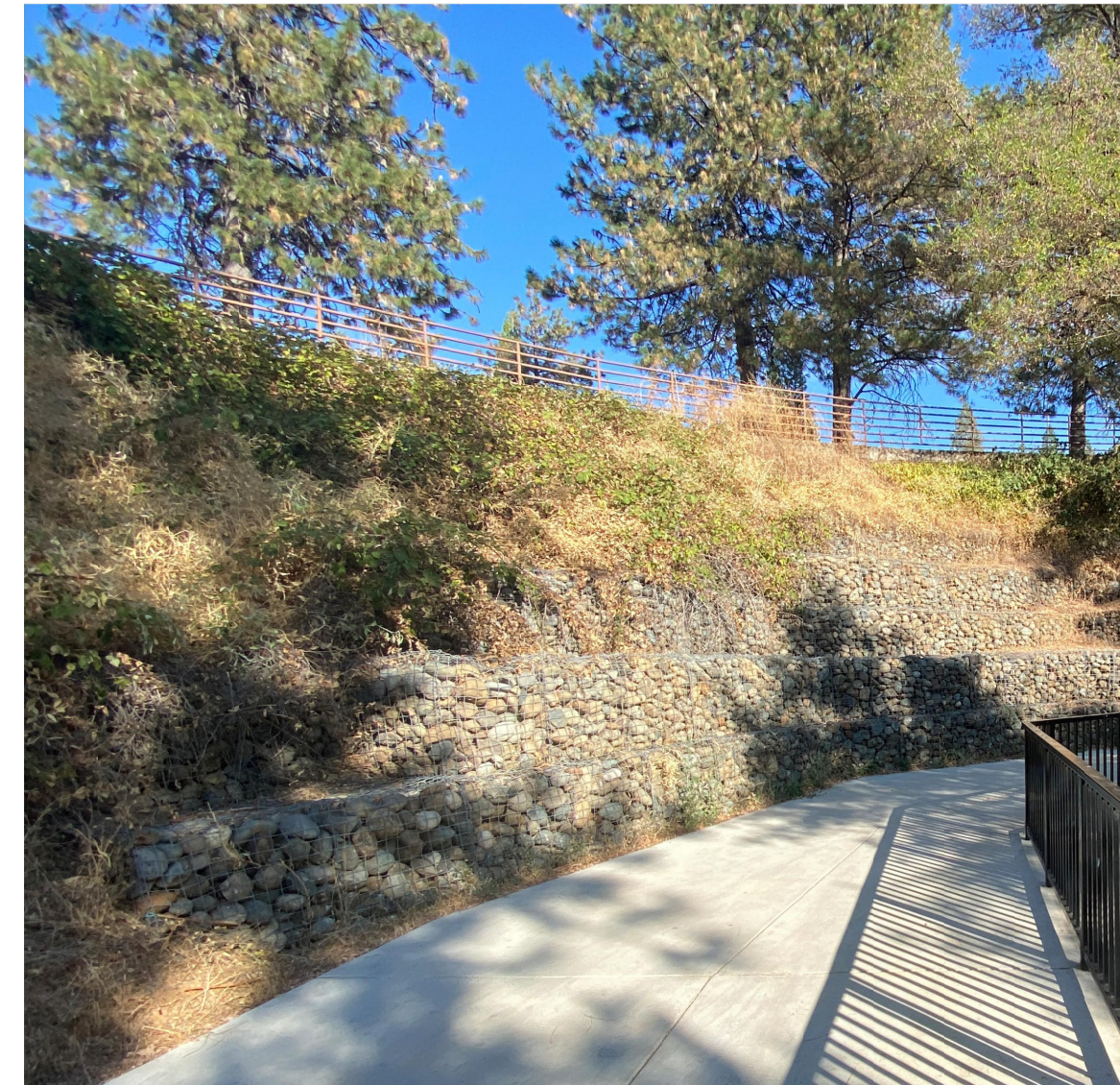
EXISTING GABION WALLS AT NORTHSTAR MINING MUSEUM
