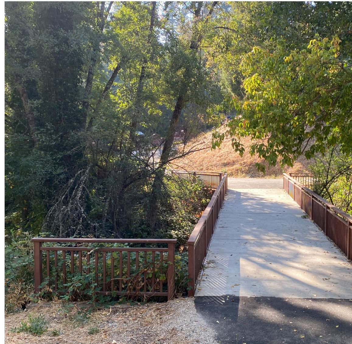
EXISTING METAL FENCE AND RAILING AT NORTHSTAR MINING MUSEUM
