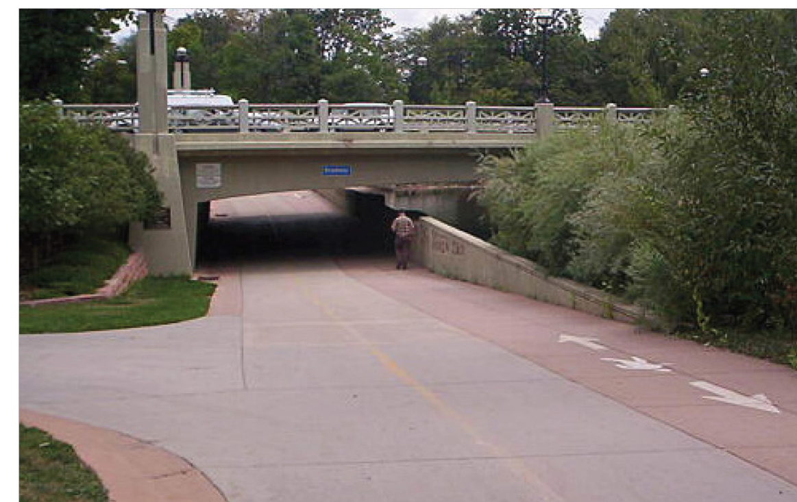
ANOTHER EXAMPLE OF PAVING USED TO REDUCE USER CONFLICT BY DISTINGUISHING SPACES FOR CYCLISTS AND PEDESTRIANS.
