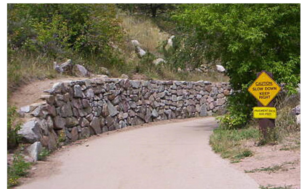
RUSTIC STONE WALL
