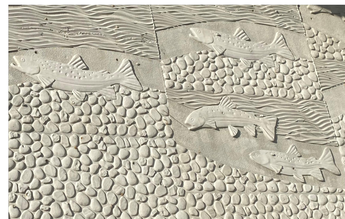
CONCRETE FORM-LINER MURAL
