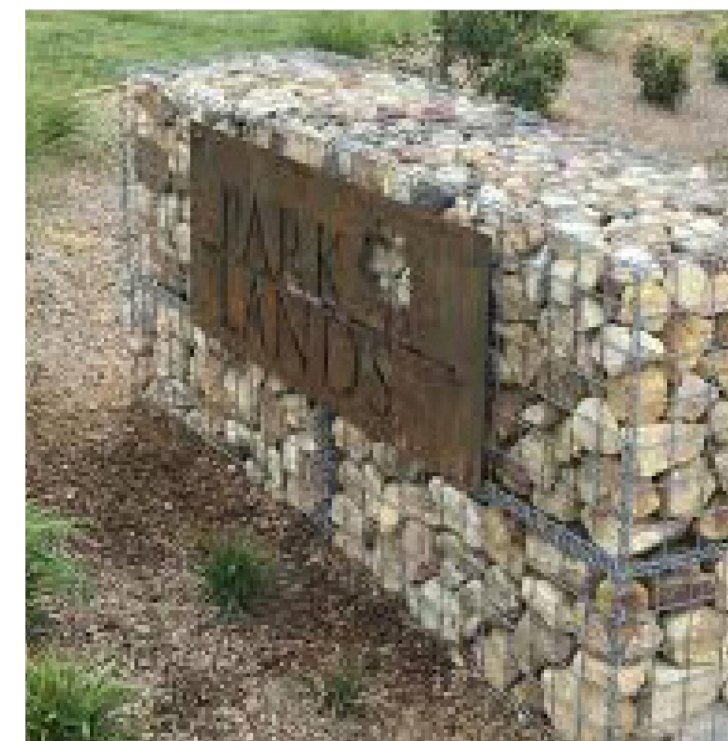
GABION WITH LASER CUT METAL SIGNAGE
