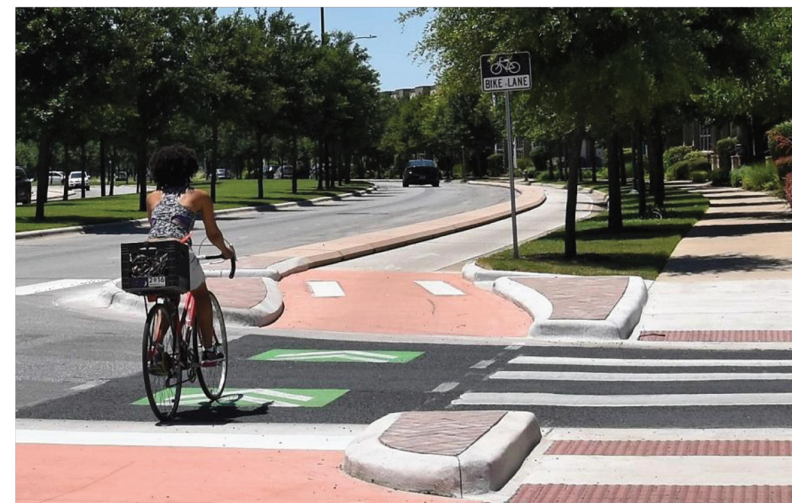
CONTRASTING PAVING COLORS GUIDE TRAIL USERS THROUGH INTERSECTIONS WITH A VISUAL CONNECTION TO THE ROUTE.
