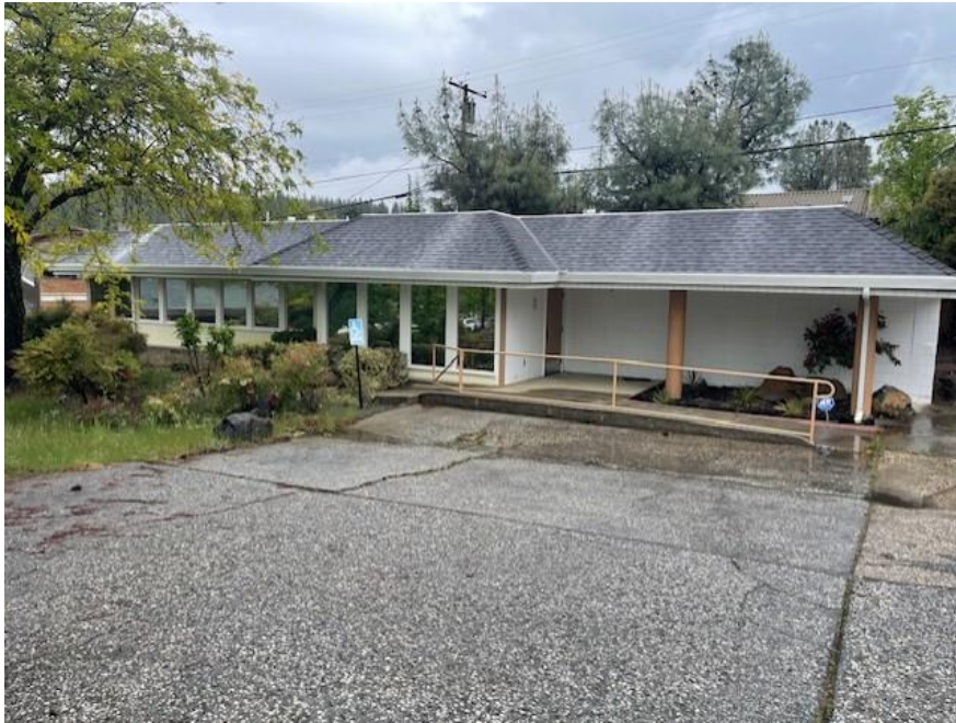
Image 1 – Front of Existing Building and Parking Lot
