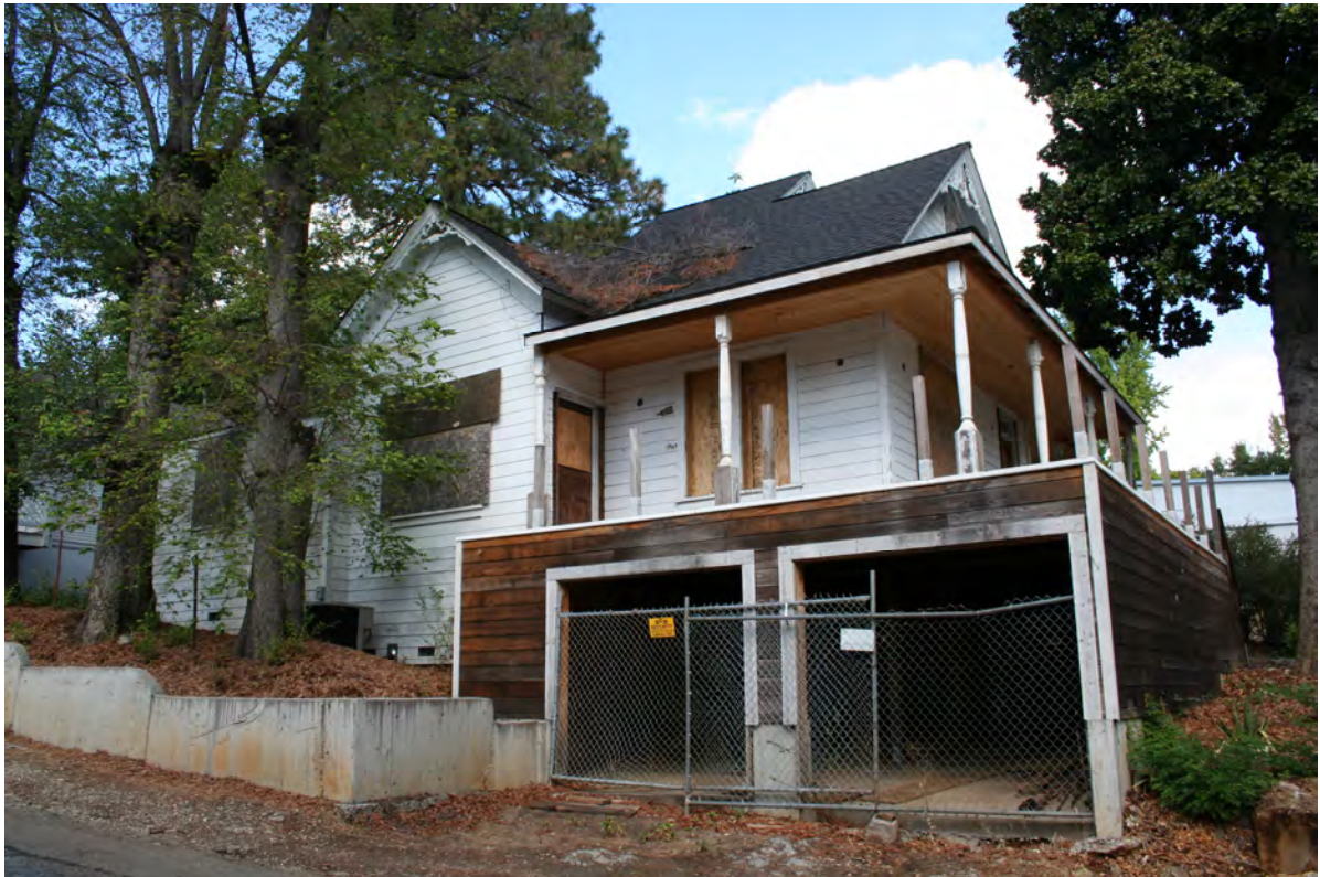
View looking north at the residence which is owned by the Grass Valley School District.
