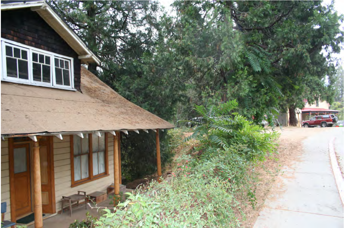
View looking south at the front facade of the residence.
