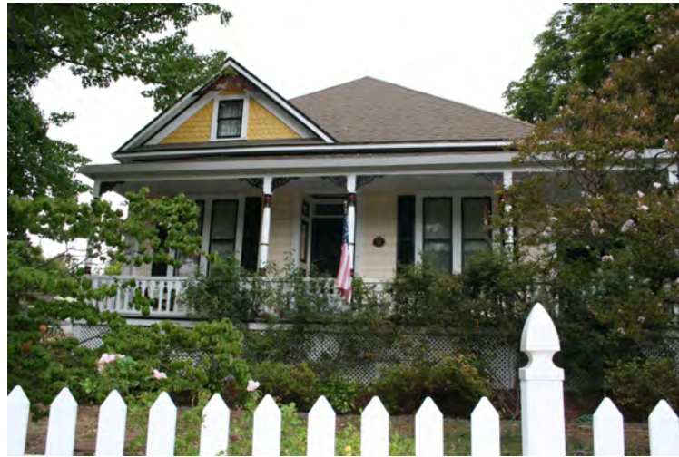
View of the front facade looking west.
