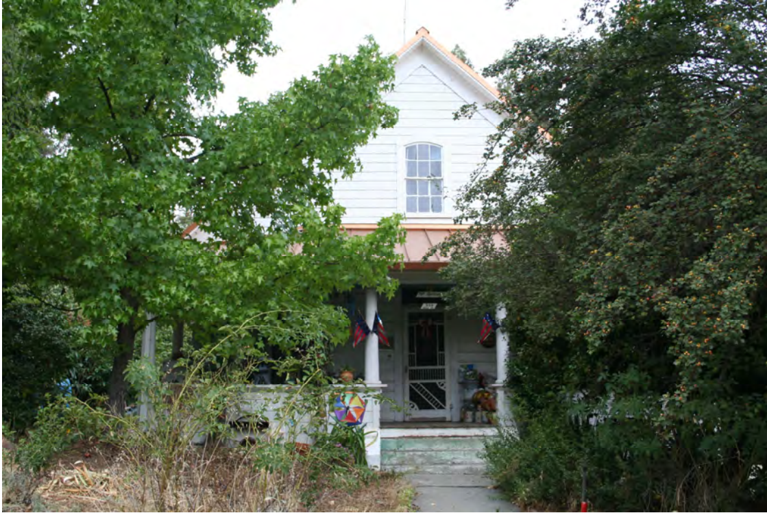
Close-up of the front facade of the residence. Note the 6 over 6 arched second-story attic window.
