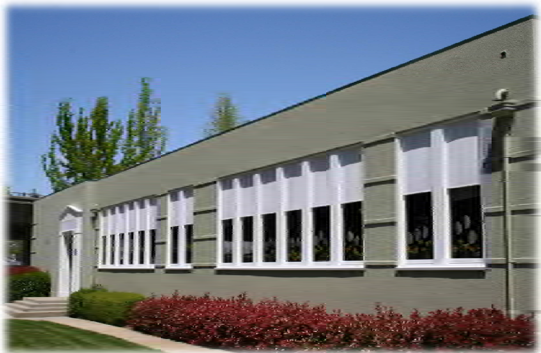
Use of a repeating ribbon type window in a Grass Valley school building.
