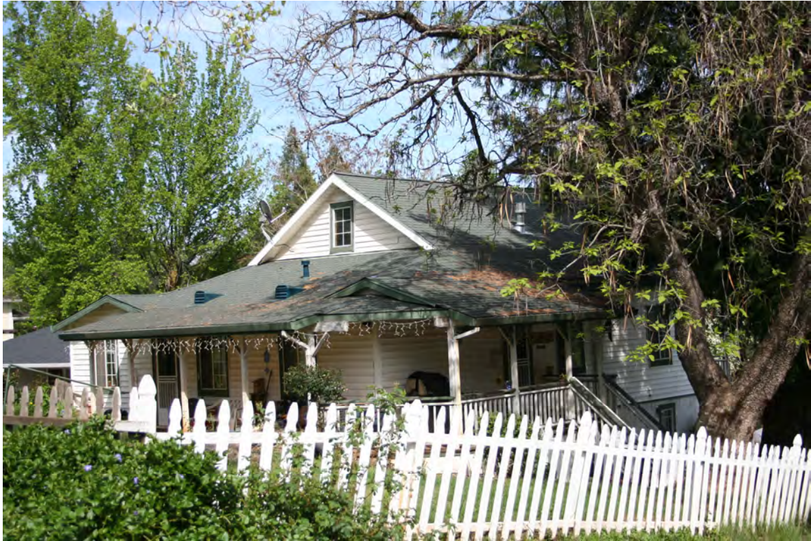
View looking northeast at the rear of the house.
