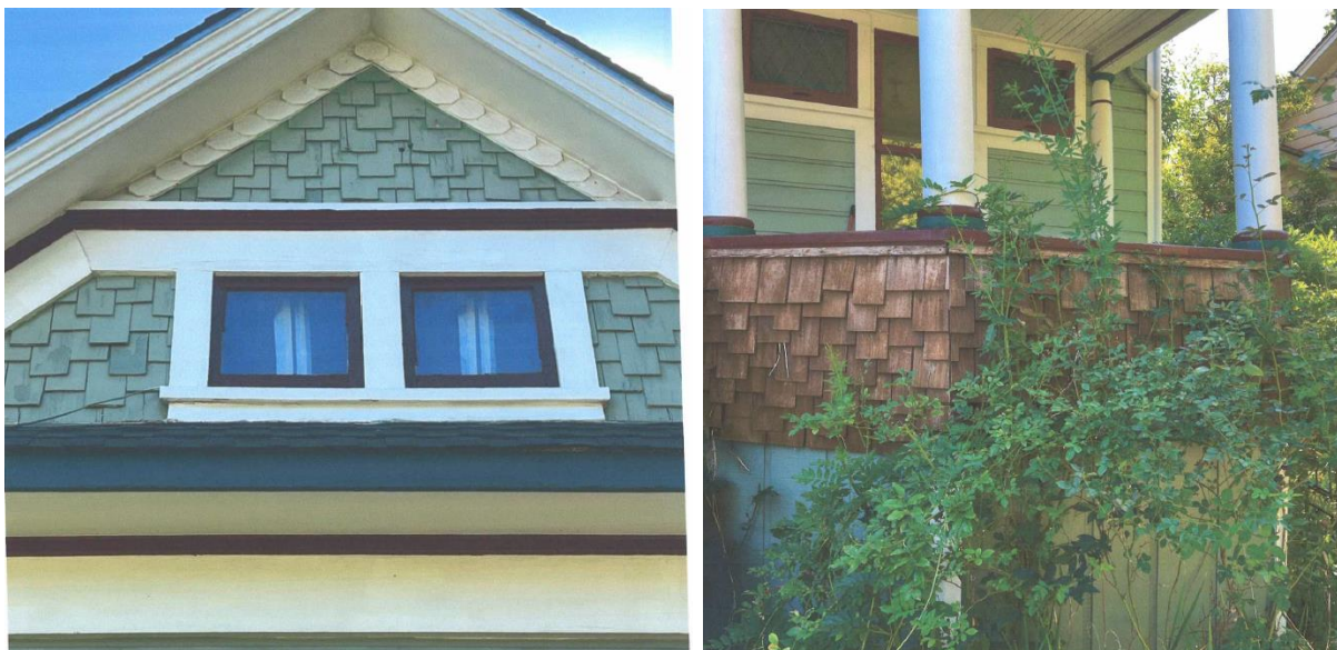
Existing Shingled Siding at 257 South Auburn Street
