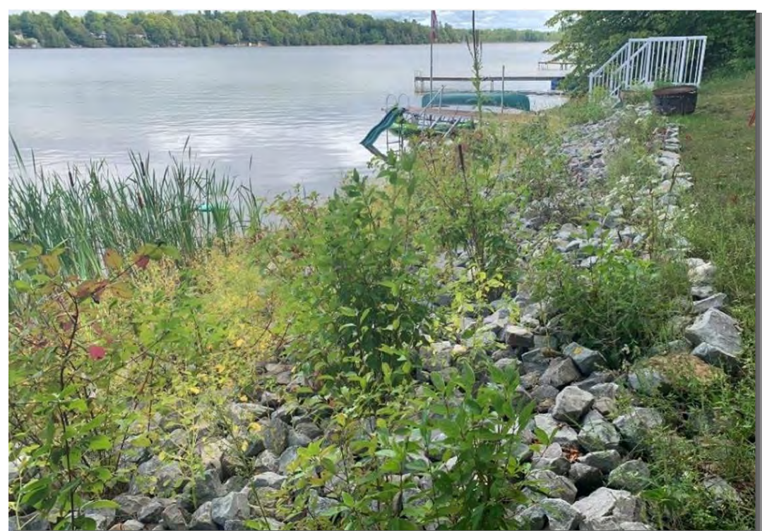
VEGETATED ROCK SLOPE PROTECTION https://watersheds.ca/wp-content/uploads/2022/06/RVCAs-Vegetated-Rip-Rap-handout.pdf
