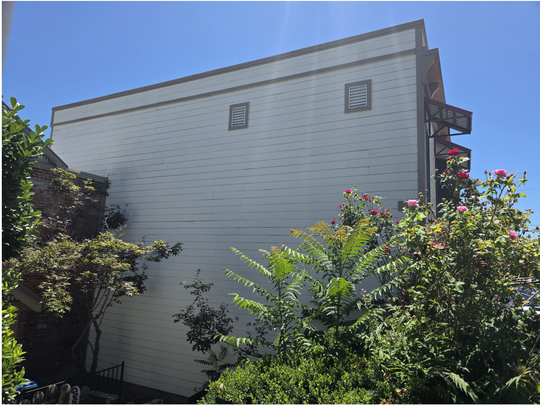
NOTE: PICTURE OF EXISTING NORTH FACADE
