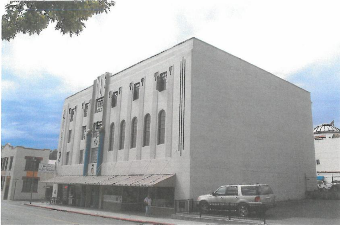
View looking south at the Masonic Building from South Auburn Street.
