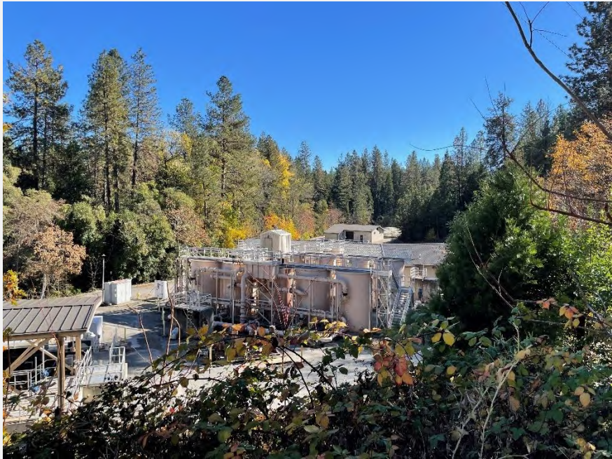
Photo 3. Dense forest adjacent to the Grass Valley Wastewater Treatment Plant, a critical City facility.
