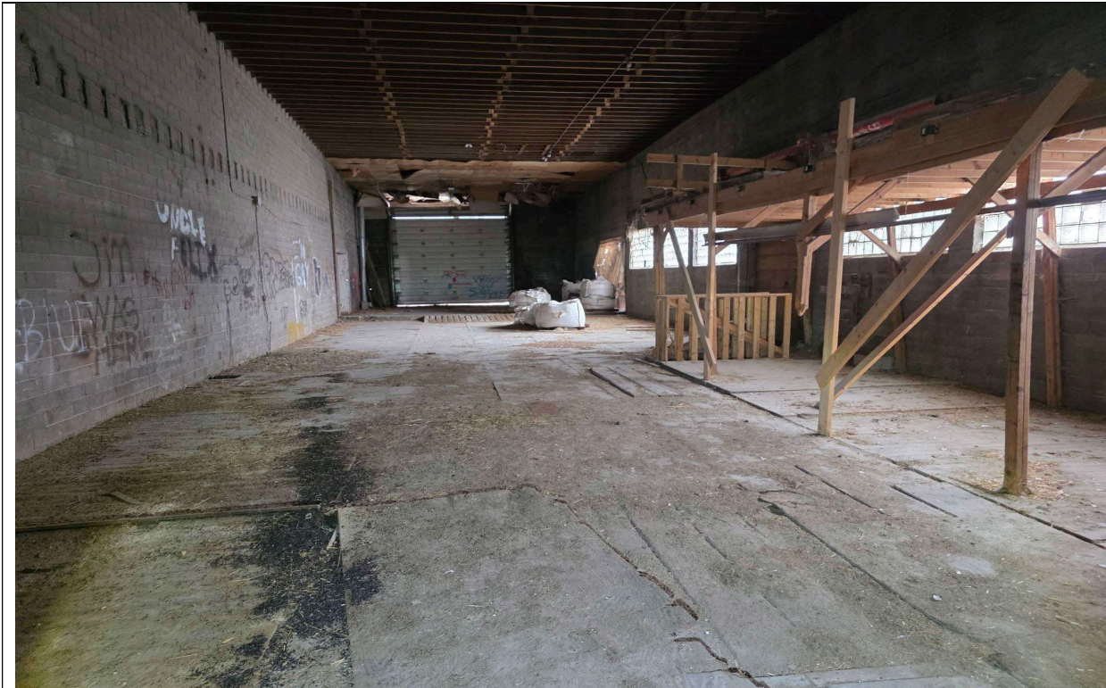
Photograph 27 Date: April 14 th , 2026 Direction: East Subject: Interior storage area and drive-through loading and unloading area in the southern portion of the Site building. Eight one-ton bulk bags of fertilizer in the southeast portion of the Site building.
