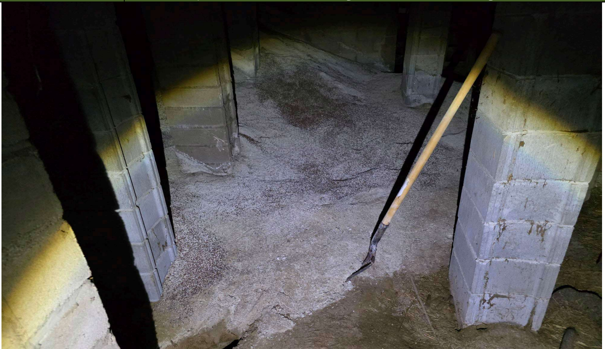
Photograph 38 Date: April 14 th , 2026 Direction: South Subject: Dirt floor area with an estimated 20-tons of unidentified fertilizer in the southwest portion of the Site building's basement bulk storage area.
