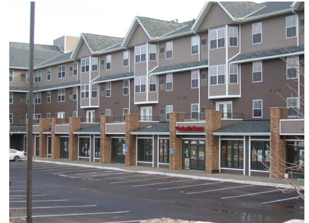
This mixed use building in Little Canada shows how housing and retail can facilitate redevelopment.
