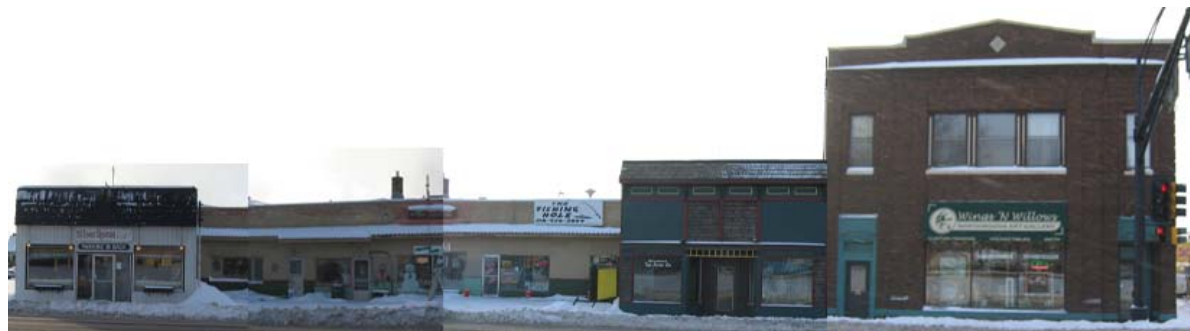
Existing building on Block 37 viewed from Highway 2.
