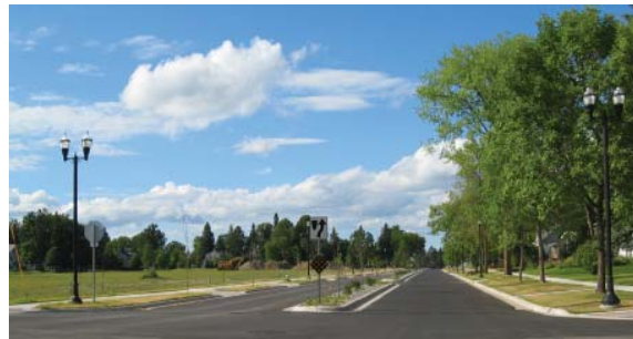
The character of the rebuilt 1st Avenue East creates a strong connection extending north from Downtown.
